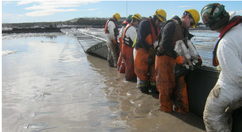
Figure 9: Seaming geotextile in one of the cells on April 1, 2011
