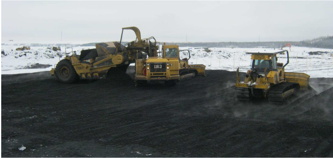
Figure 8: Photo of a CAT 631E dumping and spreading coke at the edge of a pond road
