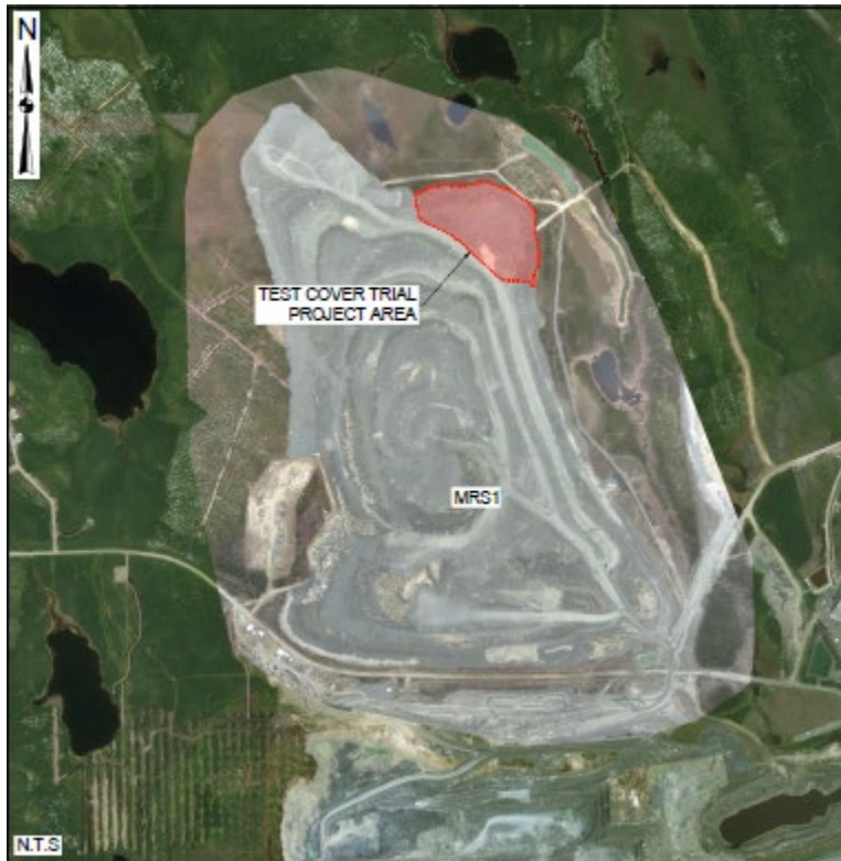
Figure 1. Test Cover Trial site location. MRS1 is approximately 2,300 m in length from north to south.
