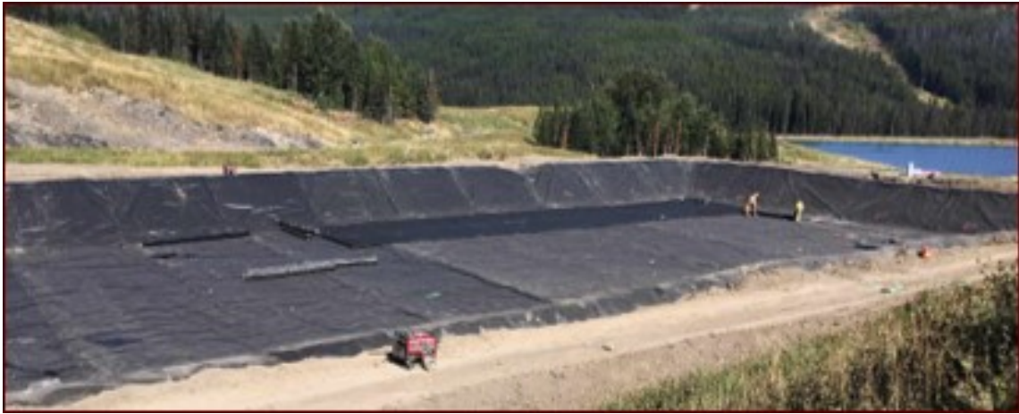
Photo 1. Reconstruction of BCR treatment cell, geosynthetic liner placement. 2017.
