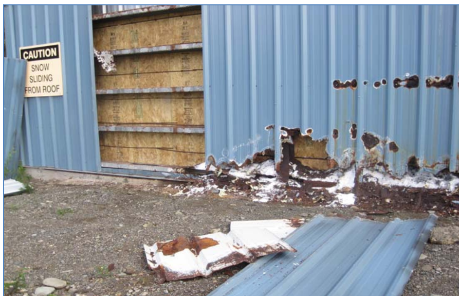
Figure 3. Photograph of ammonium-nitrate storage shed with spills to ground surface.
