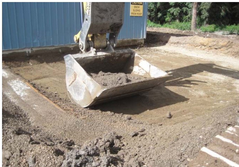
Figure 4. Remediation of Soil at the BX Facility
