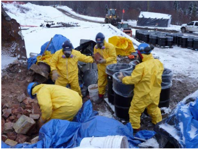
Figure 2 Preparing roaster soot & brickwork for off-site disposal
