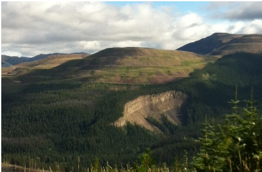
Figure 3. Waste rock dumps are set back from a failure in bedrock, ensuring long-term stability of the site.
