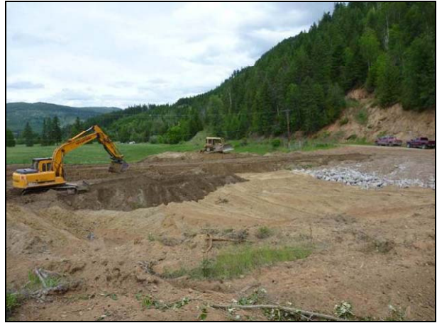
Plate 27. Backfilling tailings pond.
