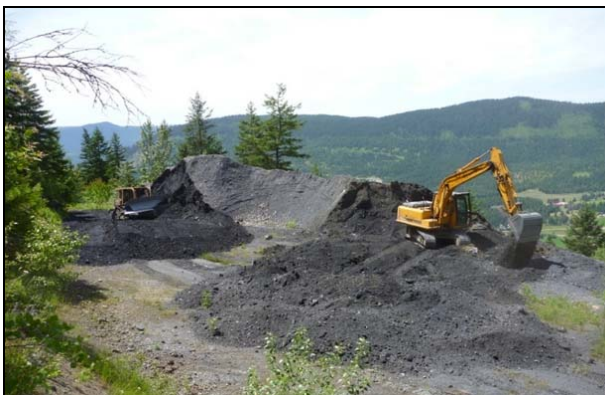
Plate 24. Spreading waste rock piles.
