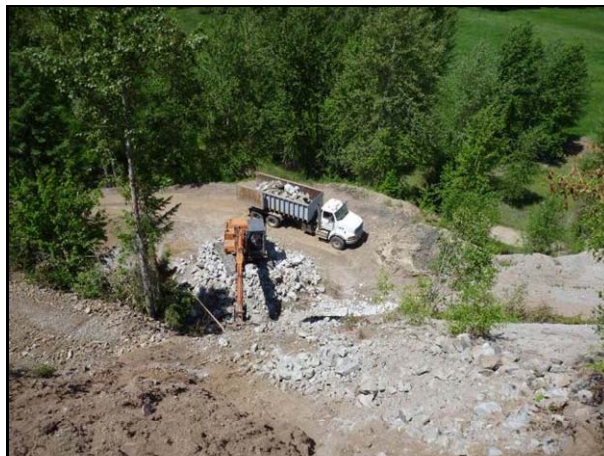
Plate 14. View of mine site from above with loading of broken concrete.
