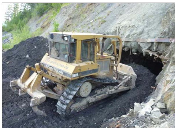
Plate 18. Backfilling of upper adit.
