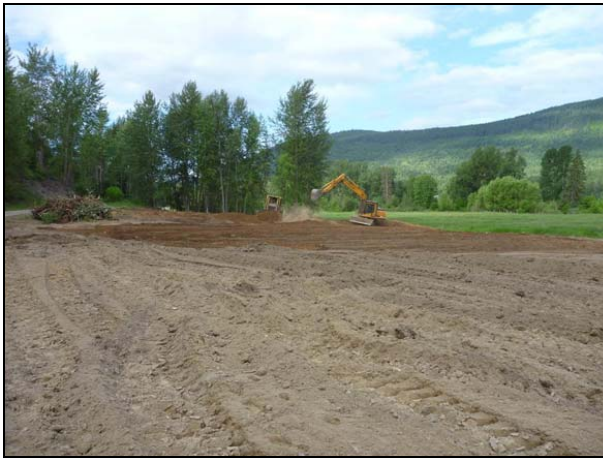
Plate 28. Backfilling tailings pond.
