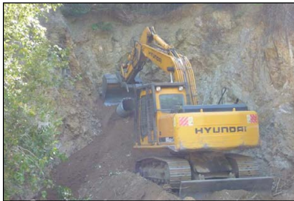
Plate 21. Backfilling of middle adit.
