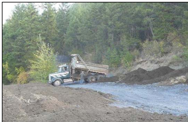
Plate 25. Spreading topsoil over waste rock.
