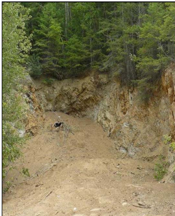
Plate 23. Regraded and backfilled middle adit.
