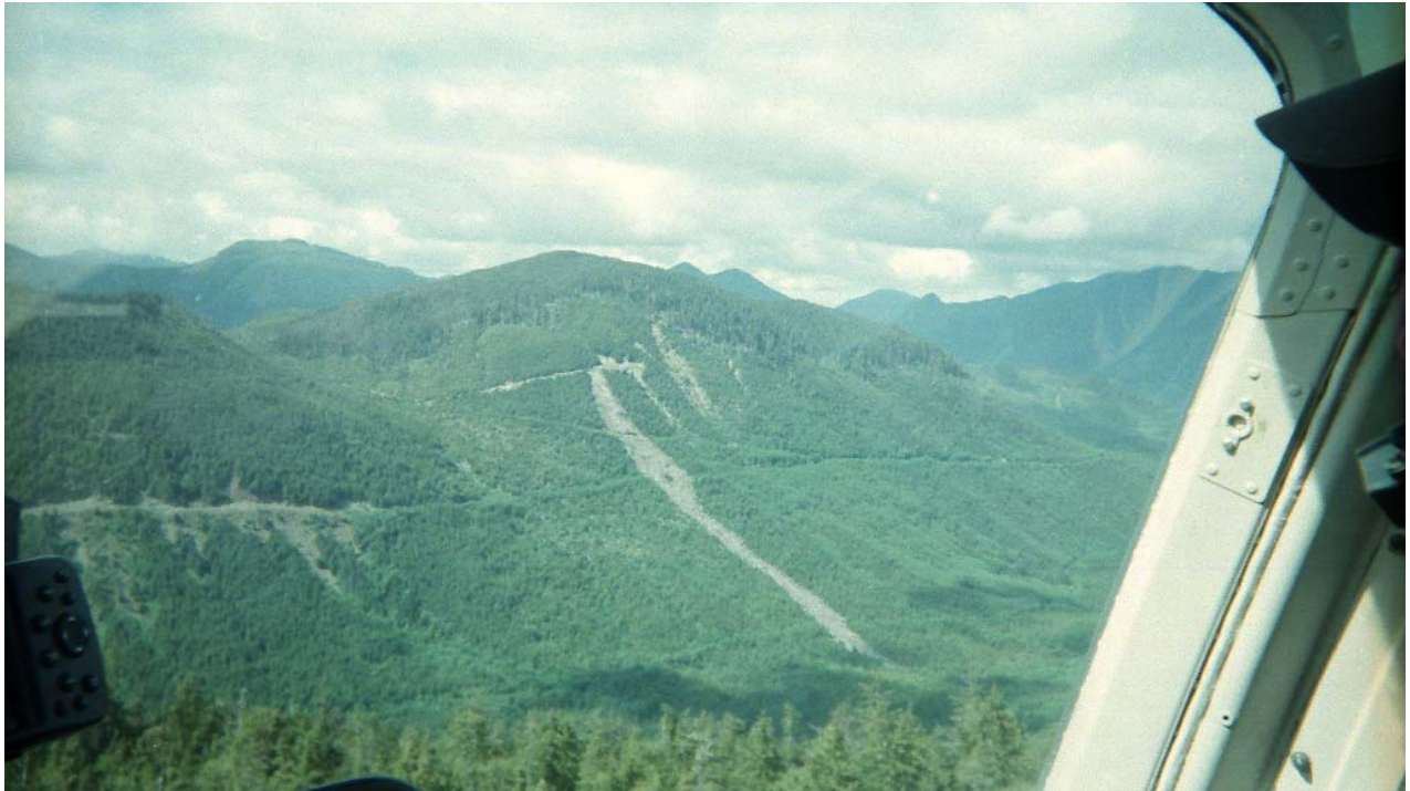
Photograph 1: A large landslide initiated at a high elevation has travelled hundreds of meters to the valley bottom impacting three other roads along the way.
