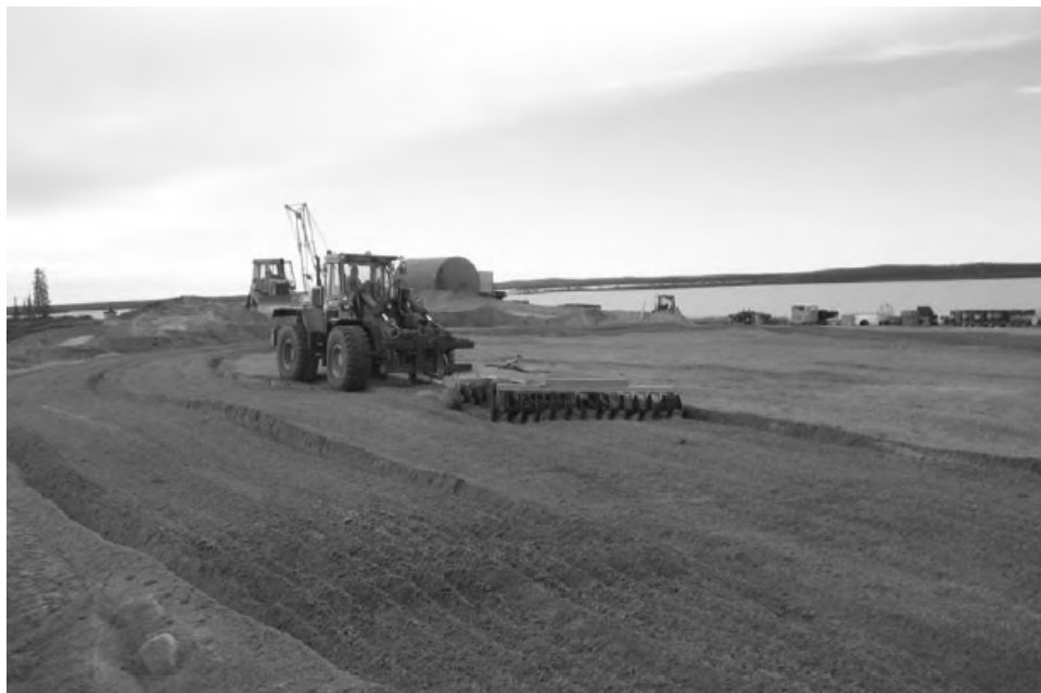
Photo 4: Discing soil on unlined landfarm
