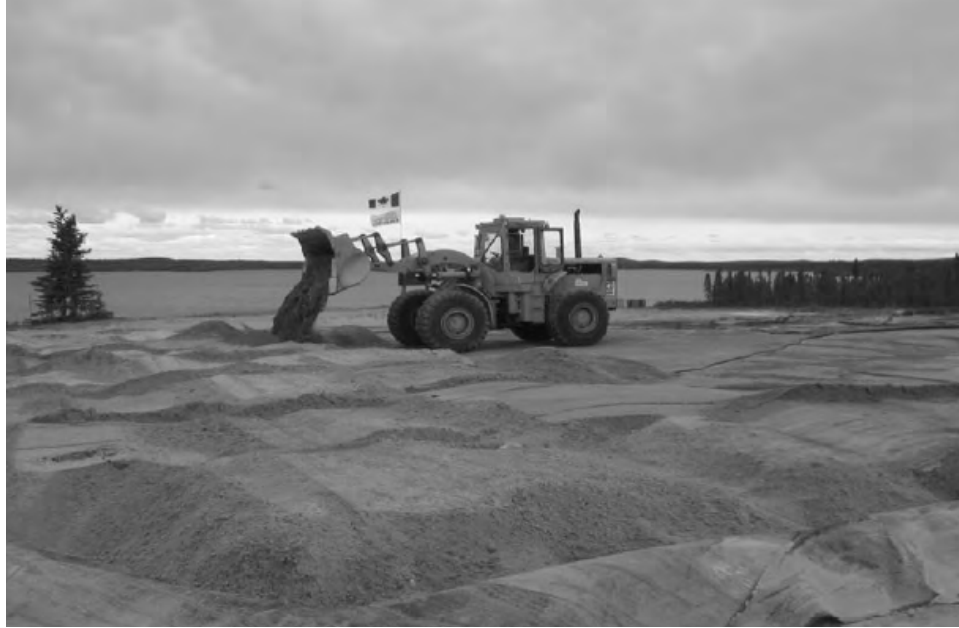
Photo 3: Spreading soil on lined landfarm
