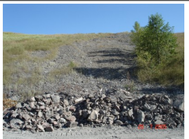
Photograph 6. The lack of vegetation cover on this strip of waste rock dump is due to a lack of till cover and the exposure of acid generating waste rocks.
