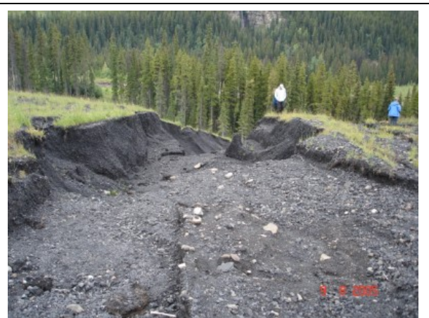
Photograph 16. Drainage from a large footwall above resulted in erosion of these coarse reject materials.
