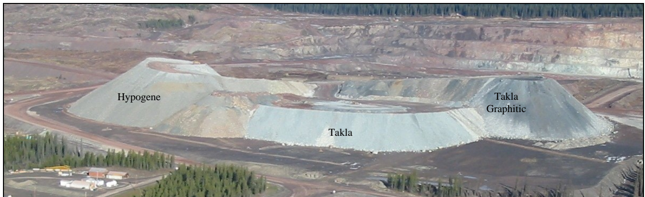
Plate 1: Low Permeability Ex-Pit PAG Dump (Showing Drainage Control And Collection Pond)
