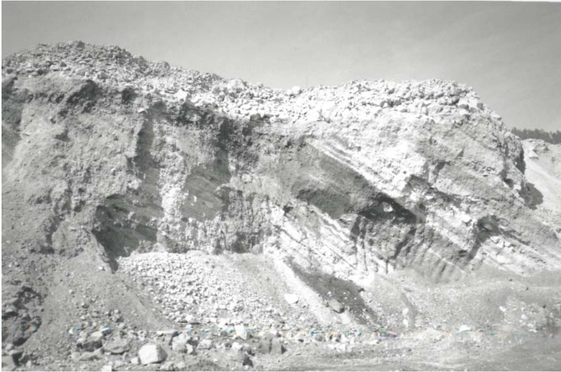
Figure 1. Dipping, layered structure visible on an excavated section of the waste rock dump.
