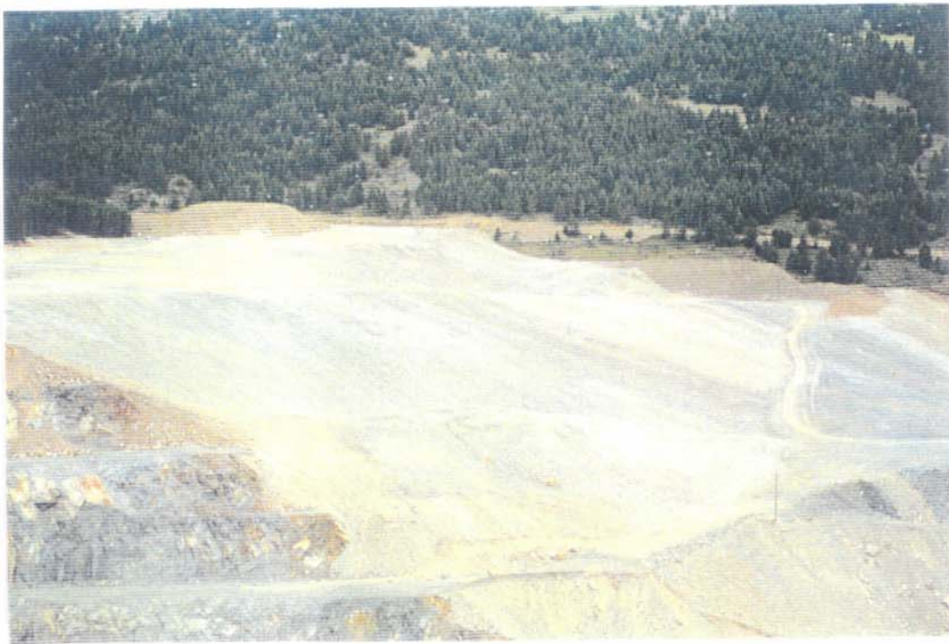
Photo 4. NORTH DUMP - Dump lifts have been resloped to angles of 18° - 24°
