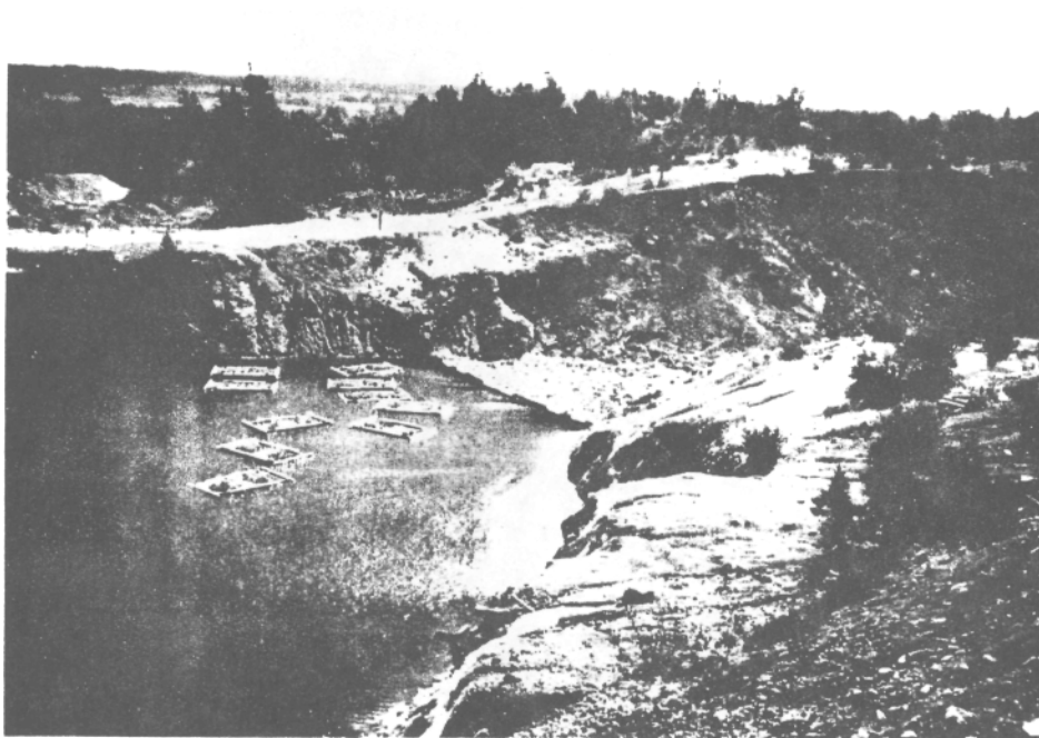
Plate 2: Acidic Pit #2 with amendment curtain, floating amendment and cattail rafts.
