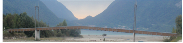
Figure 2: Suspension timber footbridge located in Fara, North-Eastern Italy, where an experimental campaign under crossing of groups of persons was carried out by the authors.
