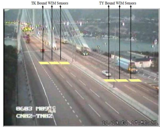
Figure 2: Layout of weigh-in-motion dynamic weigh-bridge system.
