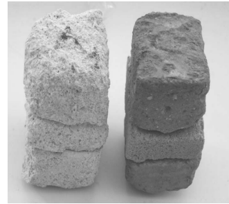
Figure 7: Appearance of deteriorated masonry samples after salt crystallization test., Cultrone et al. (2007)
