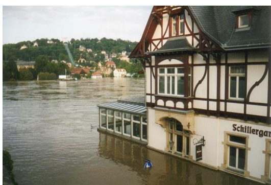
Figure 2: Flood damage in Dresden, Germany (ref: http://en.wikipedia.org/wiki/File:Schillergarten_Dresden_August_2002.jpg )
