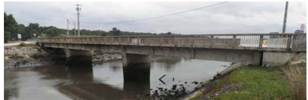
Figure 1: Lateral view of Tercenas Bridge.
