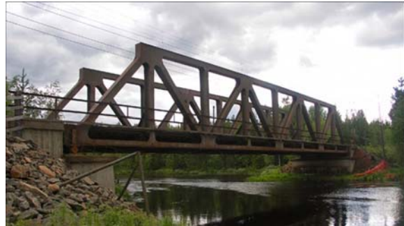
Figure 5: Lateral view of Aby Bridge.
