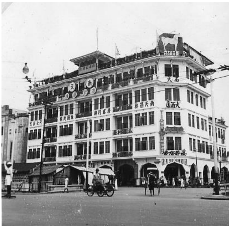
Figure 3.4 Great Southern Hotel located at the junction of Eu Tong Sen Street (余東旋街) and Upper Cross Street, Chinatown circa 1930. Photograph courtesy of the National Archives of Singapore.
