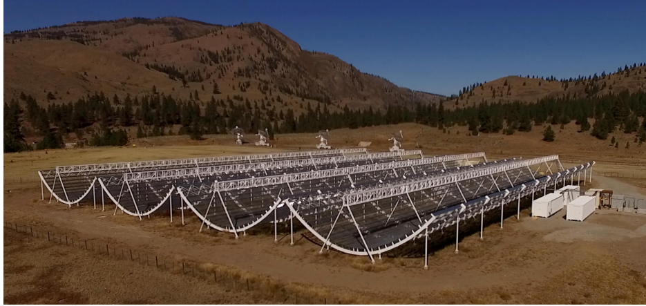
Figure 2.6: Photograph of the CHIME instrument taken at the DRAO. The metallic structures of the four cylinders and focal lines are visible, as well as the containers enclosing the X-engine. The smaller dish antennae in the background belong to a different instrument. Image credit: CHIME Collaboration [1].
