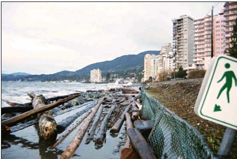
Figure 3: Centennial Seawalk after storm: path has been completely obstructed by large woody debris 20
