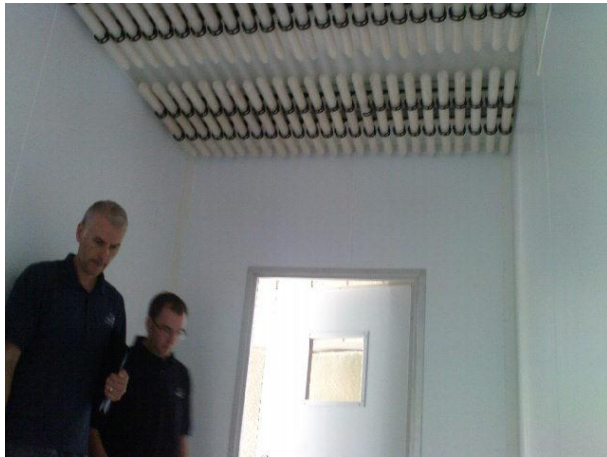
Figure 9 - Passive Cooling using Tubing Packaging. Image from pcmproducts.net
