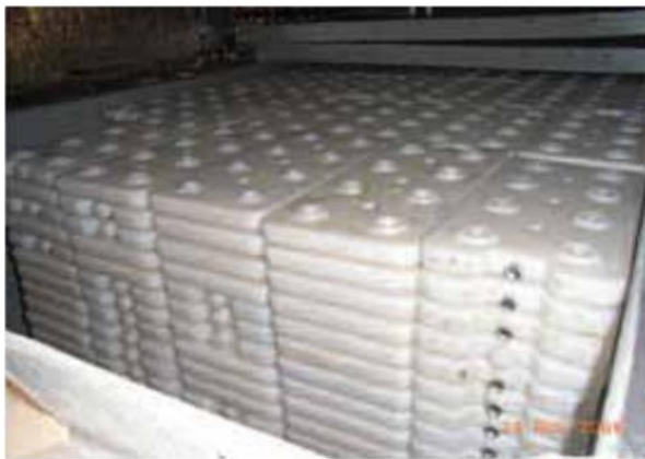
Figure 5 – Stacked Plates that form a PCM Tank. Image from pcmproducts.net
