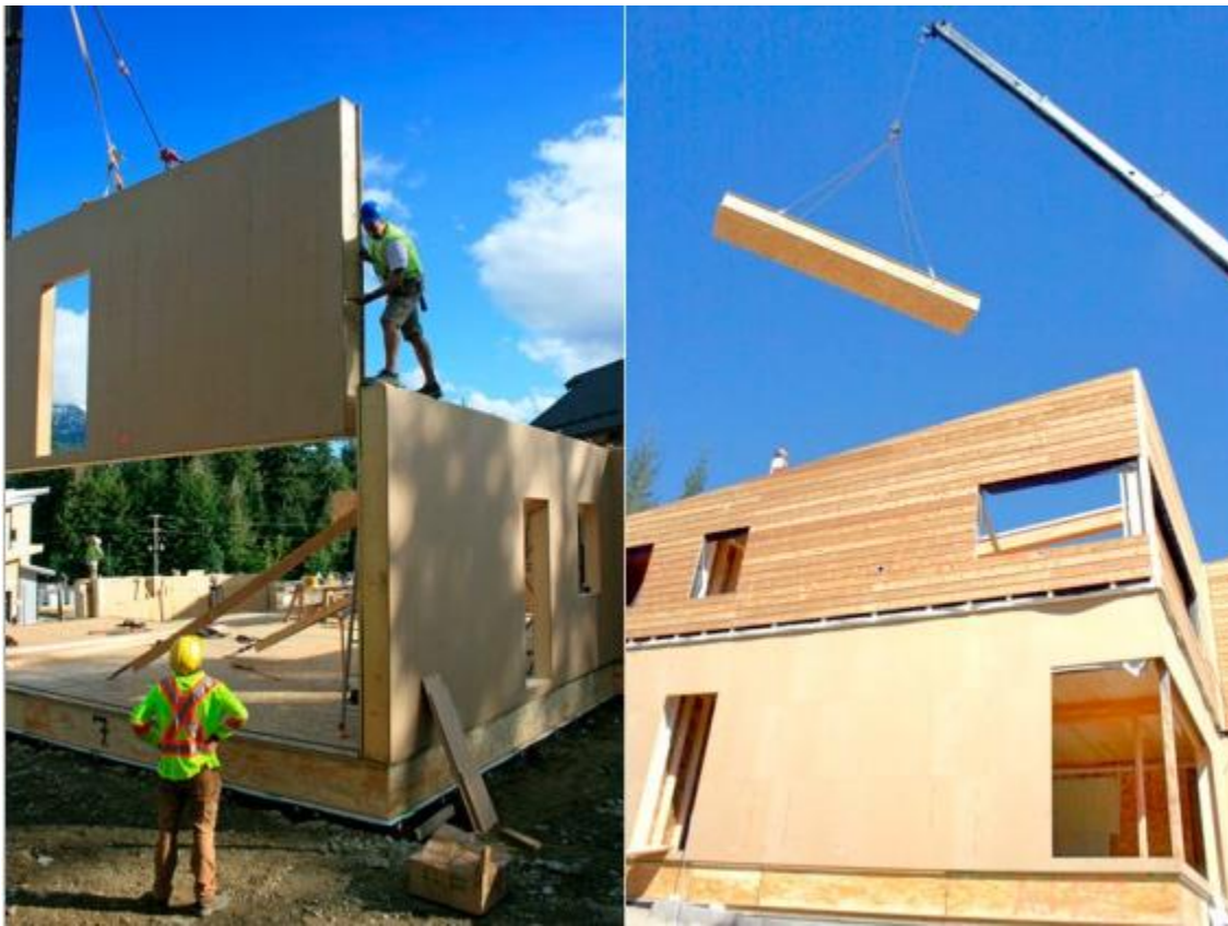
Figure 4 Panellized housing system (Preston, 2012)
