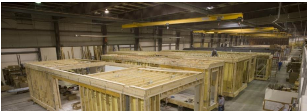
Figure 1 Pre-fabricated housing factory (Penn Lyon)
