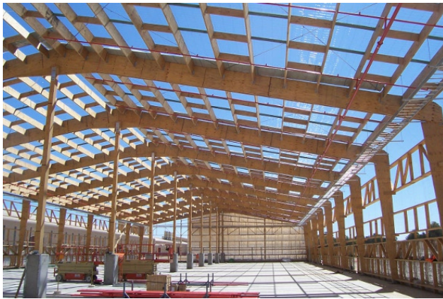
Figure 5: LVL application in Alpine MDF Warehouse, Victoria, Australia
