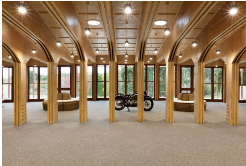
Figure 7: Application of LVL in Candlebark School Library, Victoria, Australia
