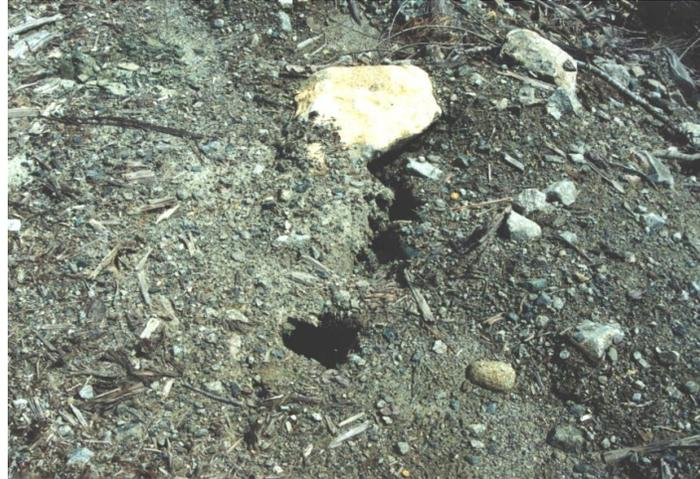
**Figure 3: Tension crack on road surface (Photo: D. Bendickson)**
