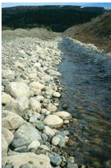
Figure 13. Faro Creek Diversion- a rock lined ditch that allows Faro Creek to flow around the Faro Mine. Modified from Faro Mine Closure Office (2009).
