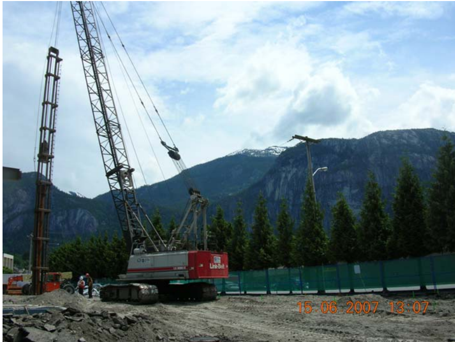
Figure III: Pile driving rig.
