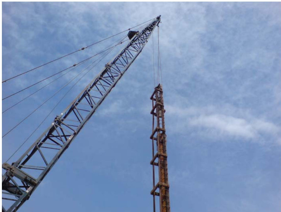
Figure II: Pile driving hammer driving pile in place.
