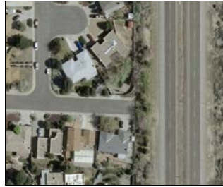
Figure 2: Routinely available airplane-based observation images for infrastructure condition assessment; this image has a spatial resolution of 0.1524-meter (6-inch).
