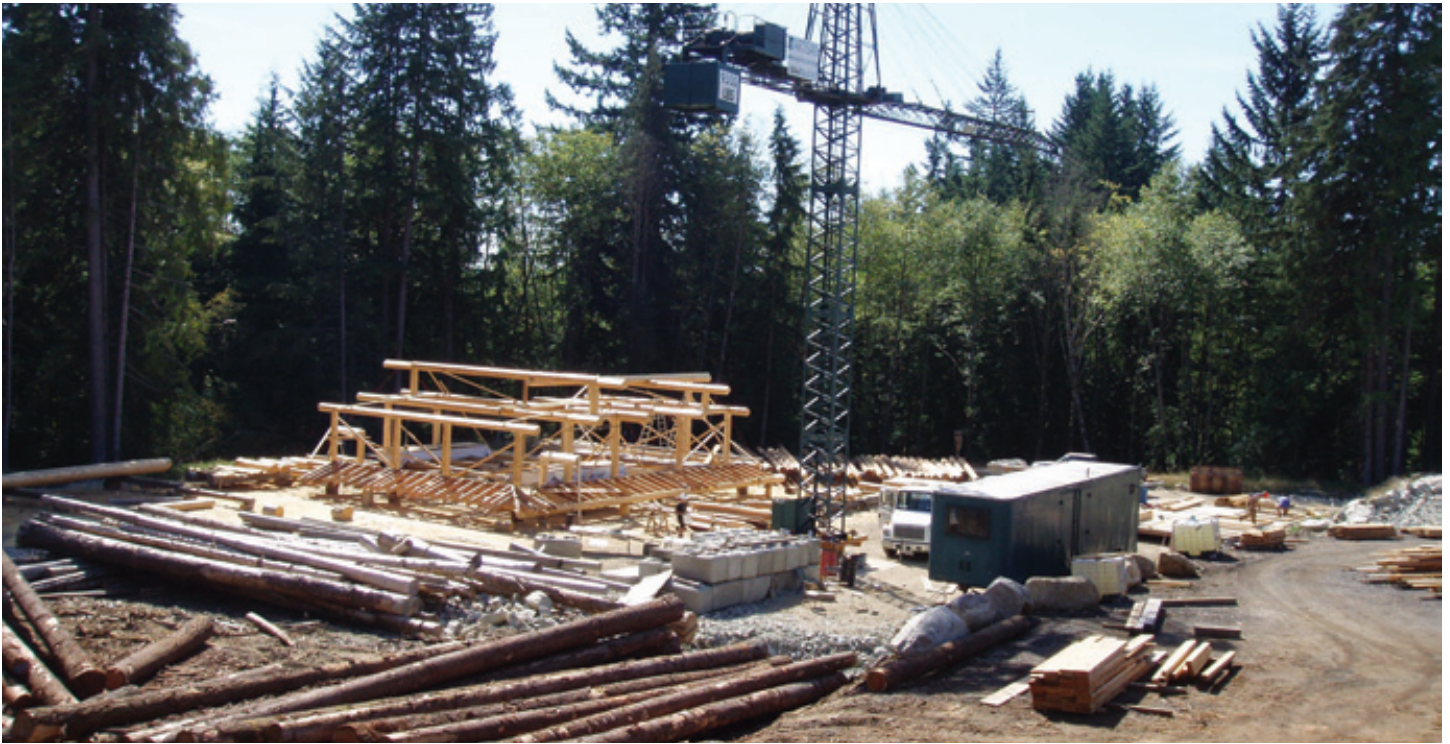
Log home construction site at the MKRF.
