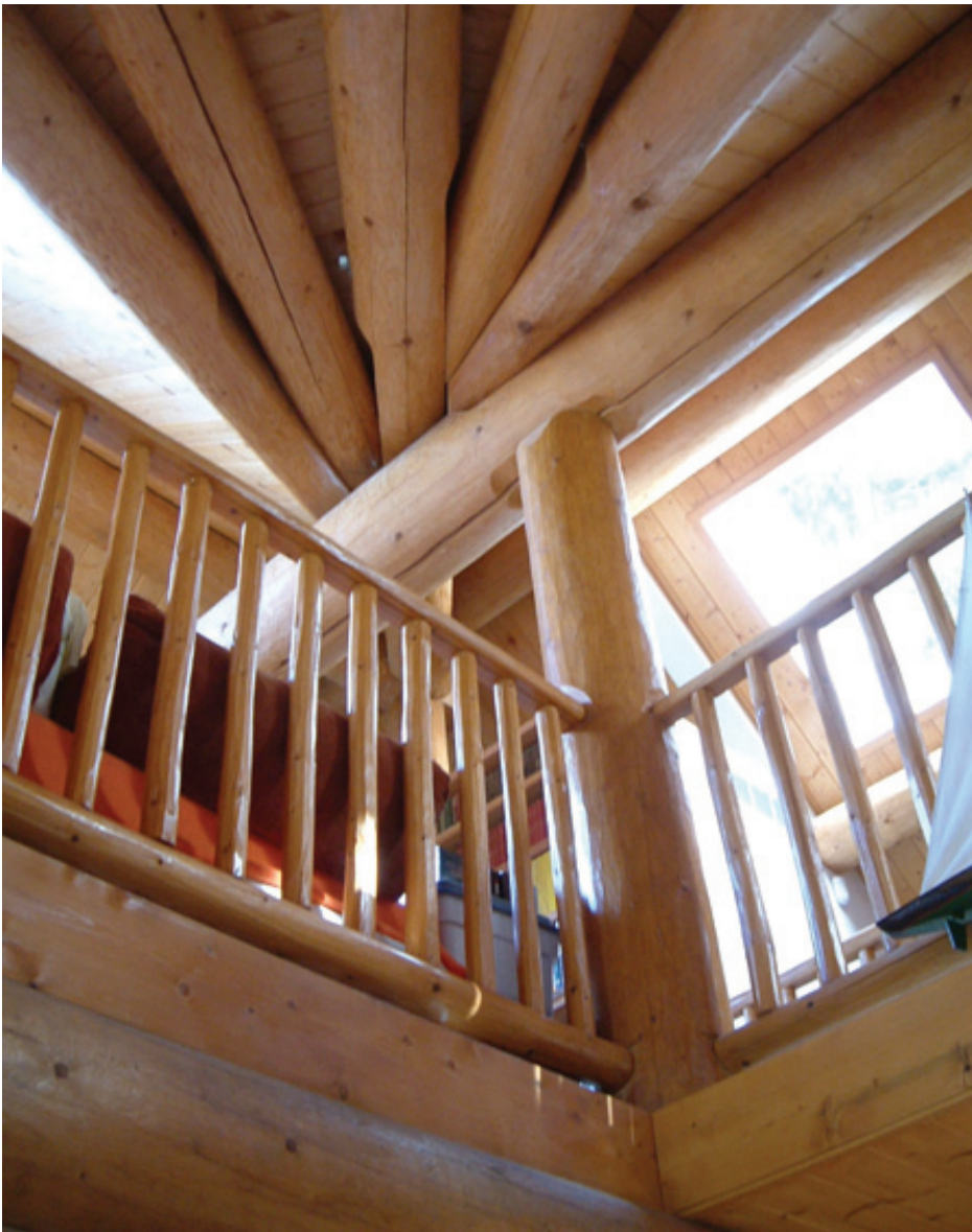
Hybrid log frame/conventional construction home.
