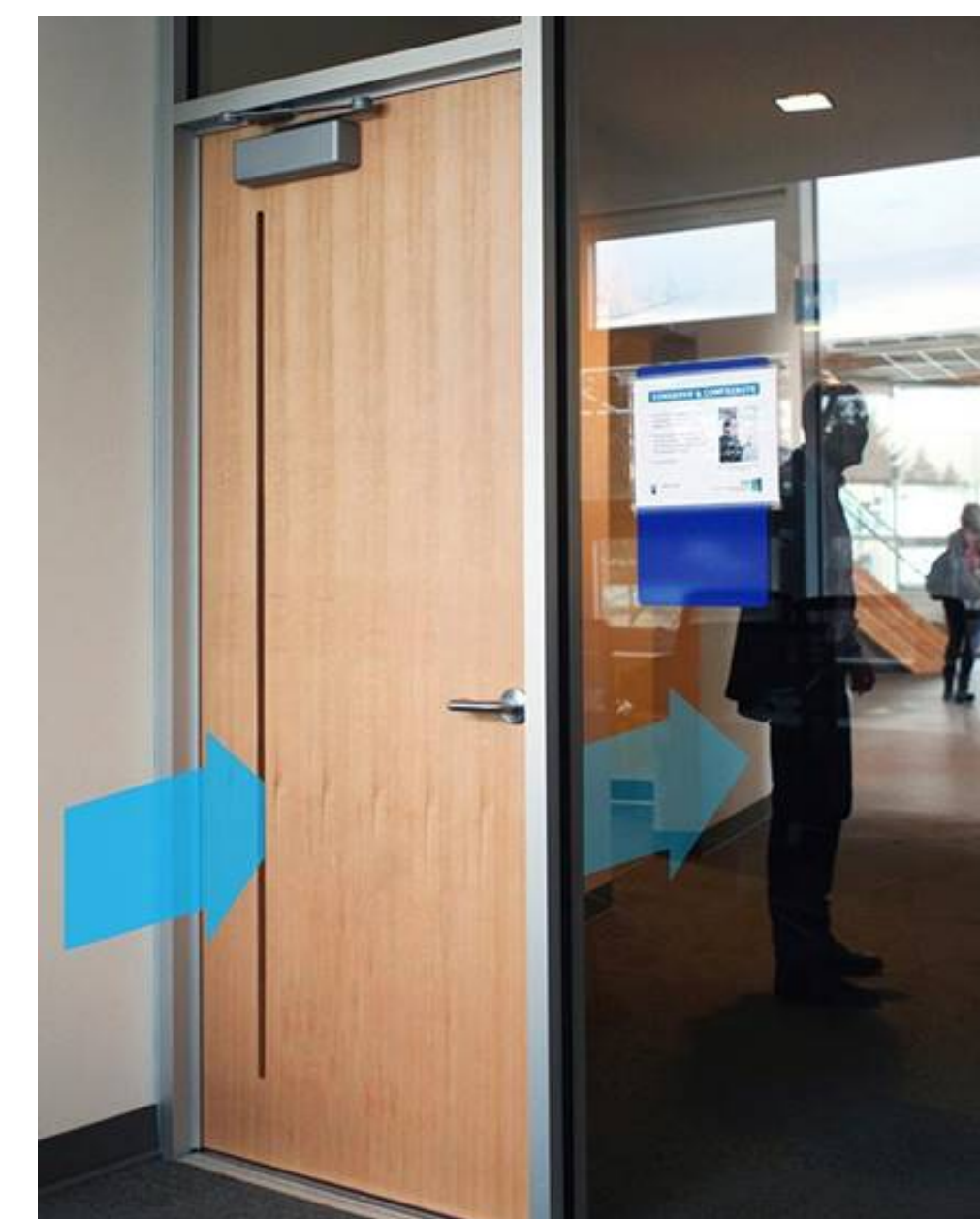
Special designed ventilated internal doors which allow the ventilation while suppressing the noise which avoid the need of using undercut doors.
