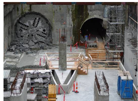
Figure 4-6: Canada Line tunnel boring machine at work in Downtown Vancouver. Source: InTransitBC (2009).
