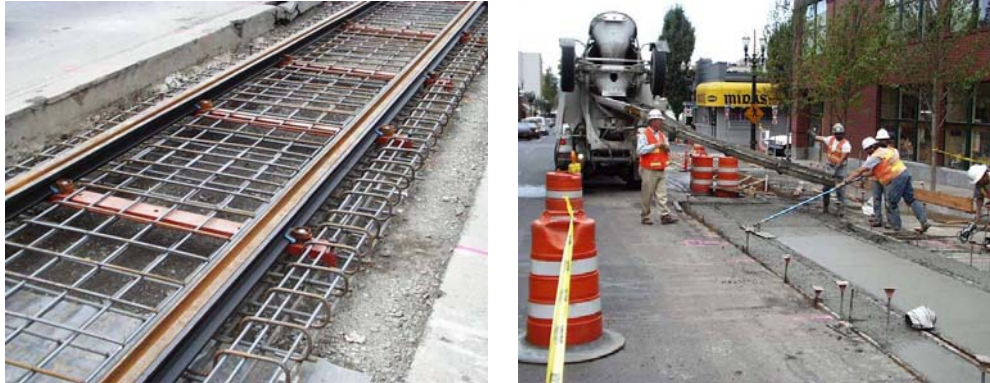
Figure 4-13: Construction of the streetcar tracks in Portland, OR. Source: APTA (2008).
