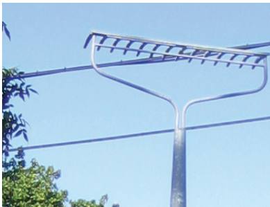
Close-up of the garden rake cyclist-activated signal "finial."
