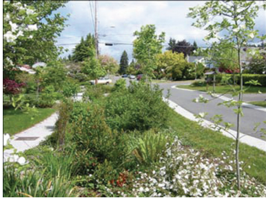
A street without traditional curbs allows stormwater to drain into planted beds at the street edge (Seattle Public Utilities, 2003).
