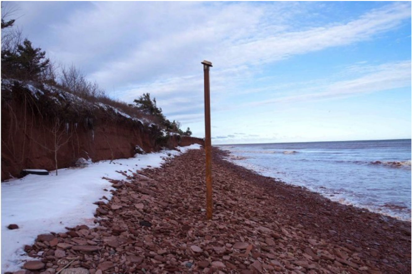
Photo 2: Exposed well due to storm surge erosion December 21, 2010 by D. Jardine.
