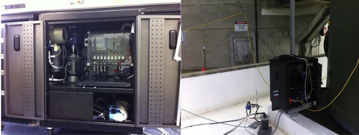
*Figure 1.4 Online dissolved sulfide monitoring system and its field installation. (reprinted from [6] with permission from Elsevier)*
