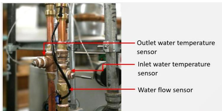
**Figure B-4: Sensors installed in water lines**
