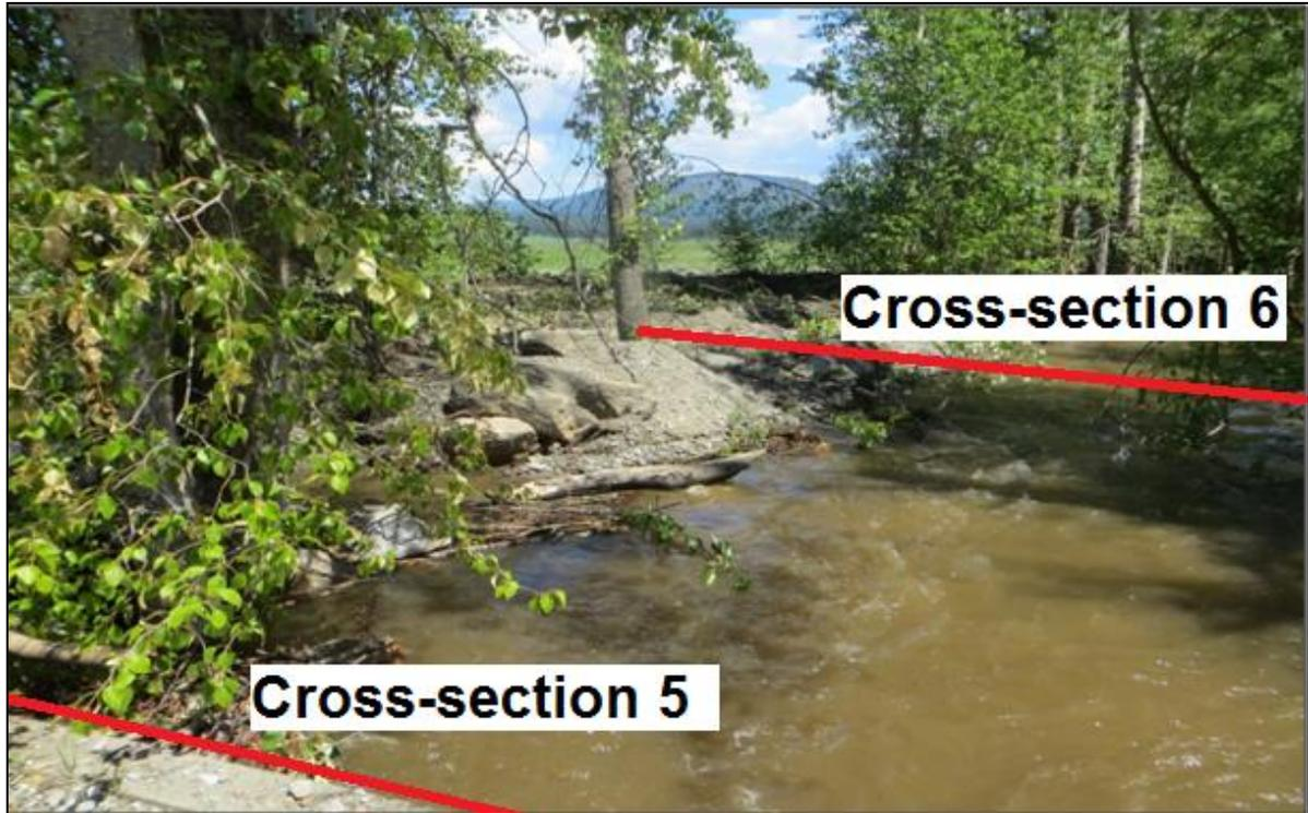
**Photograph 5. Cross-section 5 looking upstream to Cross-section 6 post emergency dredging May 28, 2017 showing the right bank dredge spoil (Photograph: L. Hettrich).**
