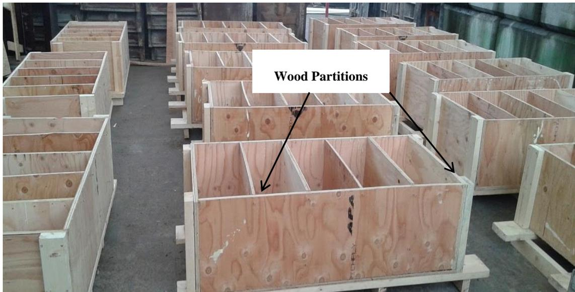
Figure 3.7 Prepared set of formwork with partitions
