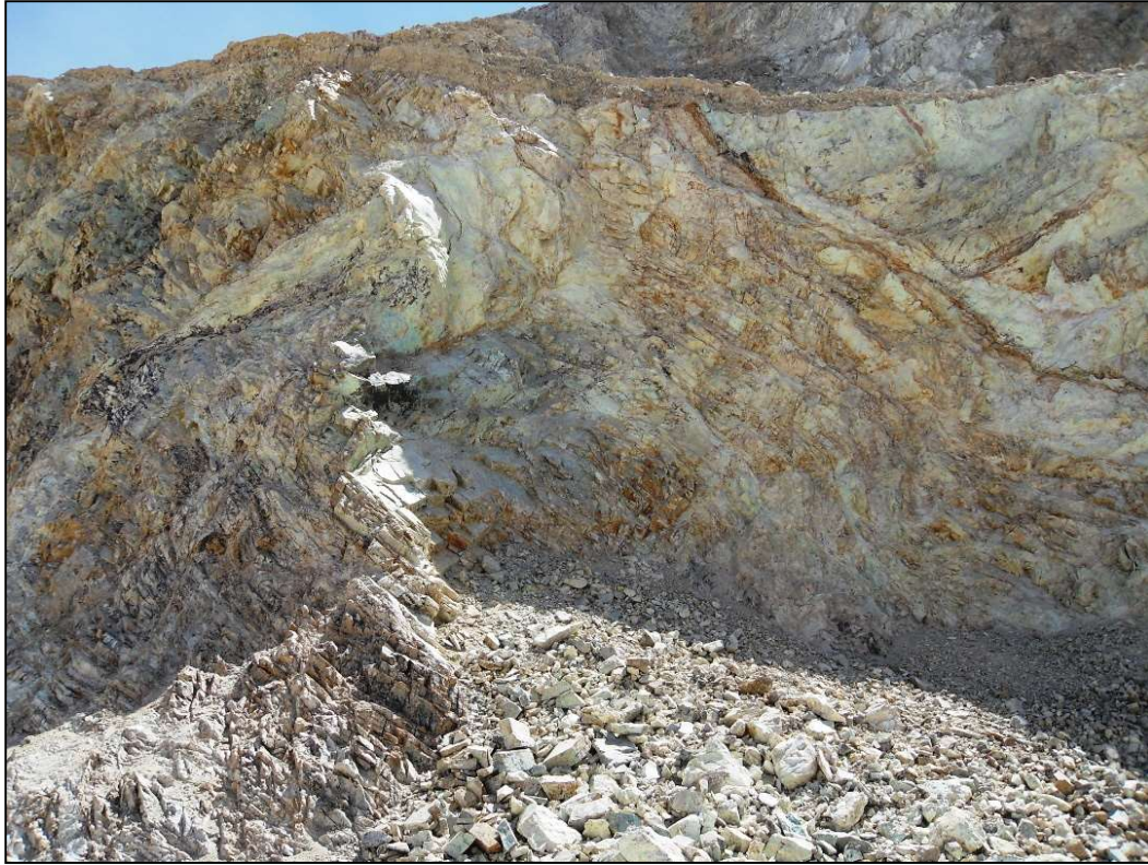
Figure 3.8. Bench excavated in Heterogeneous Leached Zone (HELZ). Brown colors corresponds to abundant Iron Oxides and Hydroxides. Note the high degree of fracturation of this geotechnical unit.
