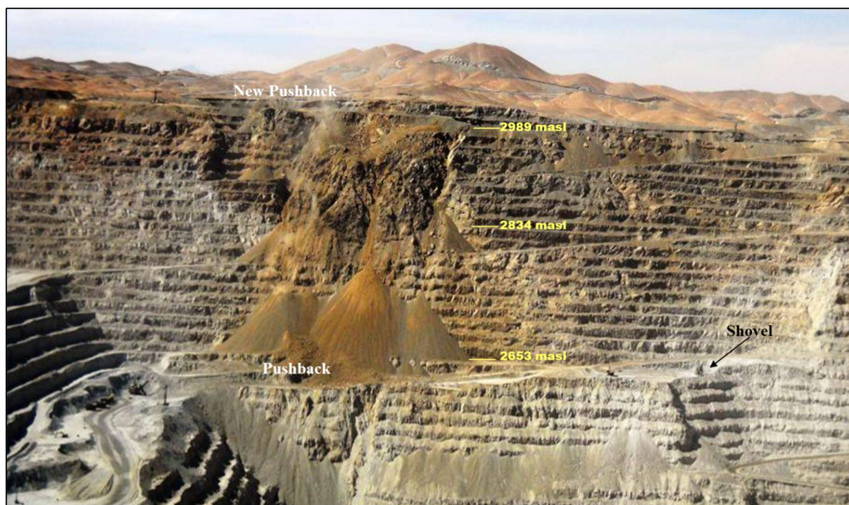
Figure 5.1. Inter-ramp slope failure on which back analysis was performed. The rupture extends approximately from 3000 meters above sea level (m.a.s.l.) down to 2830 m.a.s.l. A pushback was located on top of the failed rock mass and 180 m below the toe of the breakage. A shovel is shown as scale reference.
