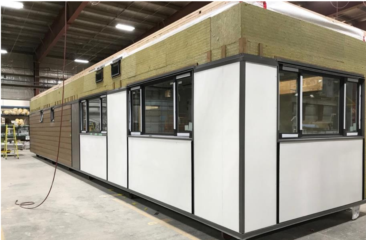
Figure 8-6 Finished module at the factory (Image source: Metric Modular)
