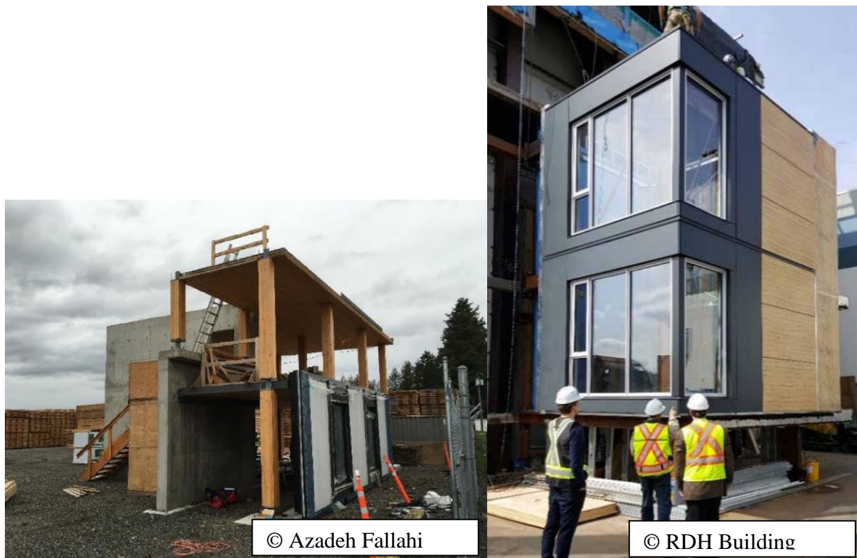
Figure 7-7 Mock-up testing (Image source: Fallahi (2017) & RDH Building Science)
