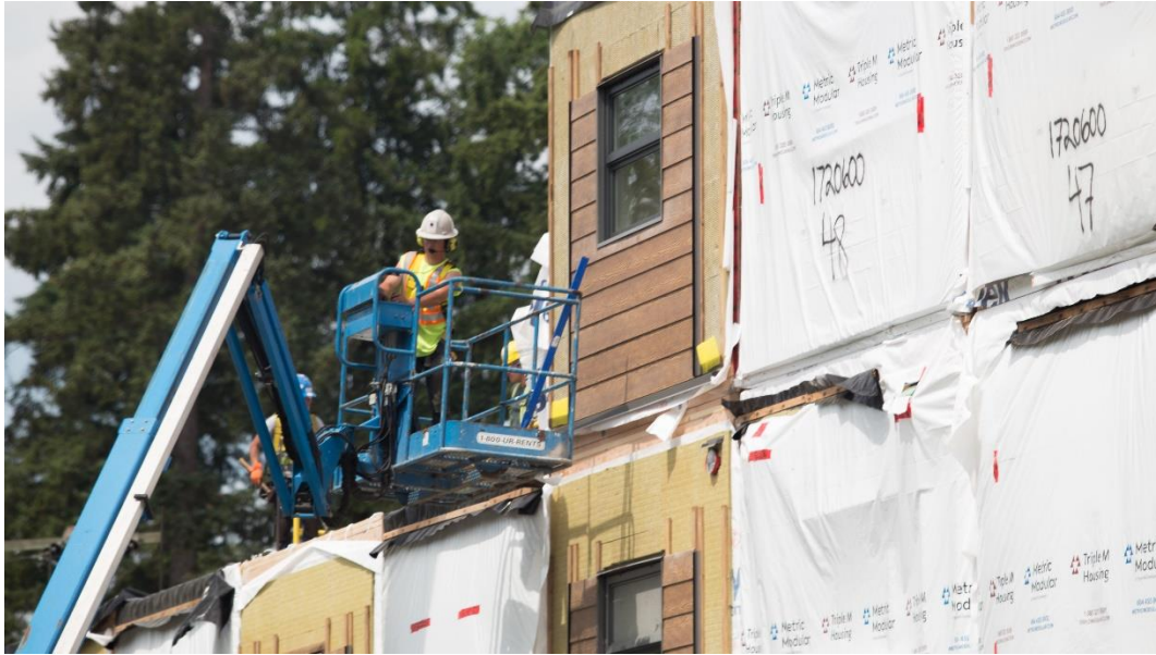
Figure 8-10 Inter-module connection process (Image source: Metric Modular)
