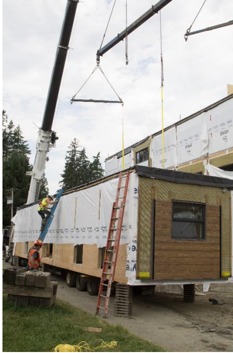
Figure 8-9 On-site installation of module (Image source: Metric Modular)
