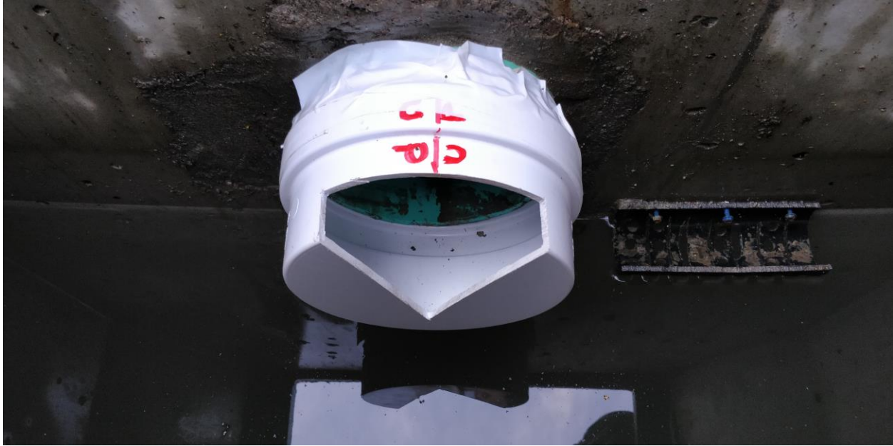
Figure 4.6: 6" PVC weir cap installed in a 6" distribution pipe inside a typical CoV CB
