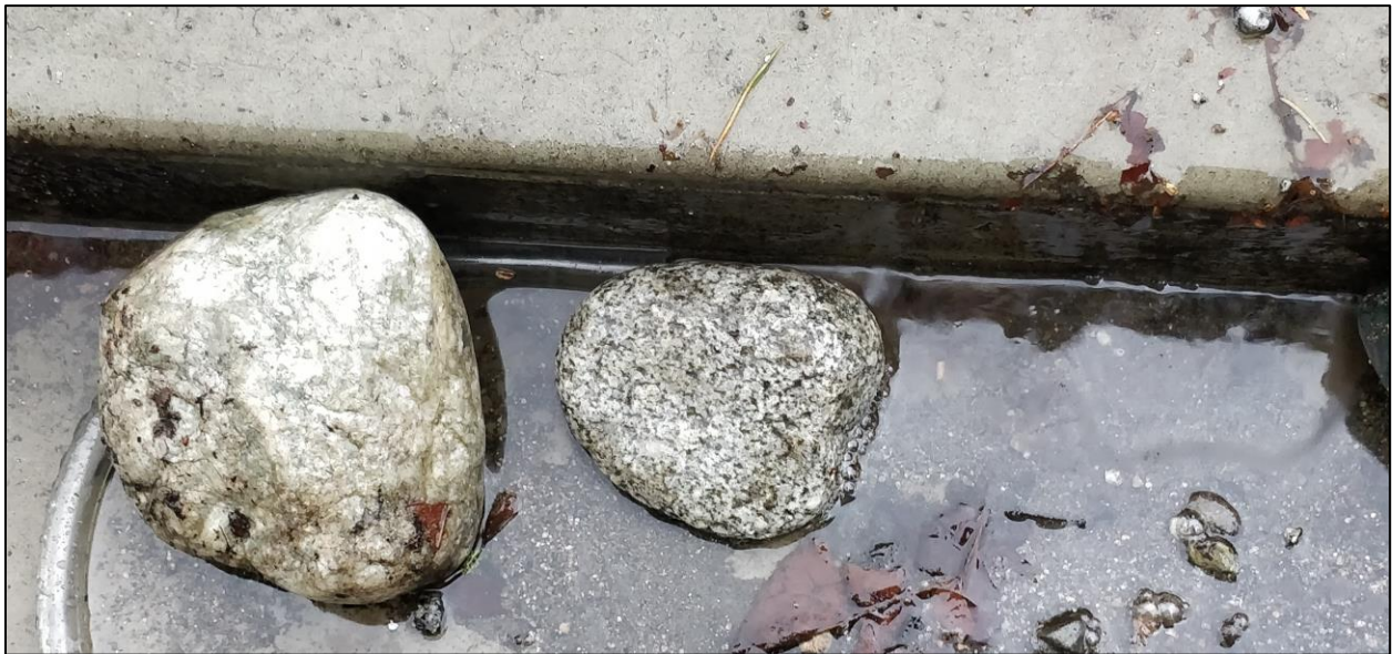
Figure 4.34: PVC tubing hose secured by rock. Rocks are also used here to pool water at the hose inlet to improve suction
