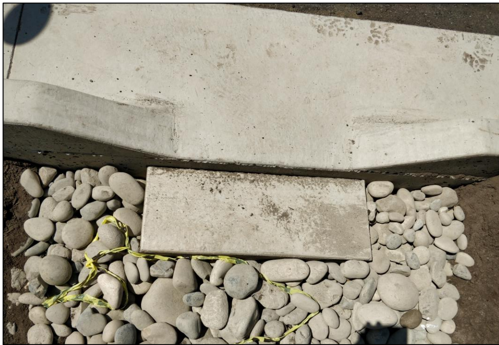
Figure 4.2: Bioswale Inlet Design shortly after being completed. Opening is flush with the street curb's gutter. Water flows into the inlet and drops into a concrete slab with the purpose of trapping fine sediment. The water is dispersed radially into river stone to disperse sediment and reduce flow speed.
