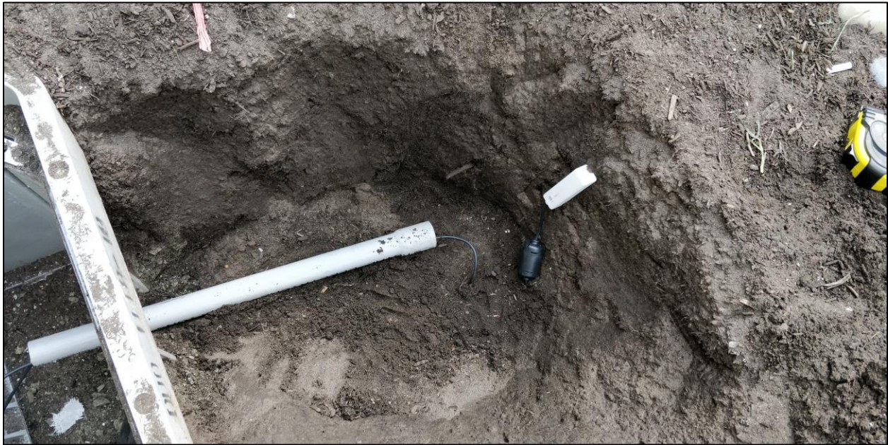
Figure 4.31: Installation of soil sensors in Bioswale 1
