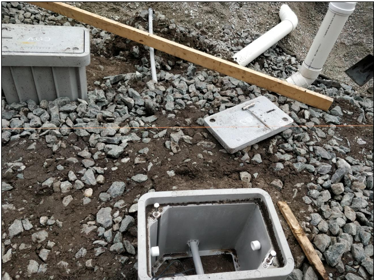
Figure 4.30: Final product. The soil sensor cables were pulled through to the valve box where the data logger installation location.
