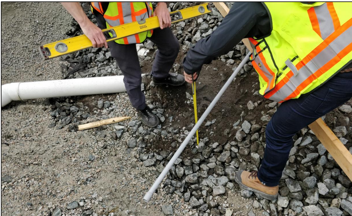
Figure 4.28: Assessment of the conditions for the soil sensor installation. The horizontal 1" PVC pipe in the picture was left by the CoV crews as a protection bridge to guard the soil sensors cables to the valve box.
