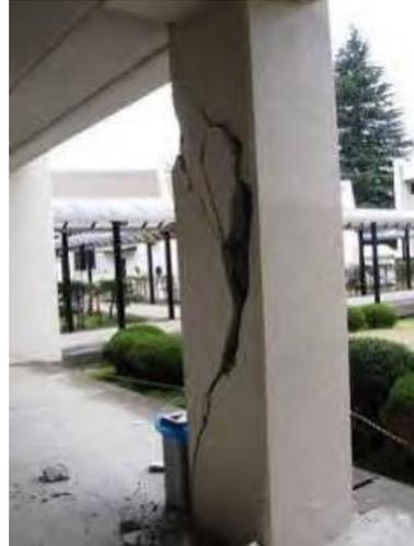
**Figure 2-20: Shear cracks on first-storey column in Sendai caused by aftershocks (Nishiyama et al., 2011).**
