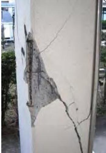
**Figure 2-19: Shear cracks on first-storey column in Sendai (Nishiyama et al., 2011).**
