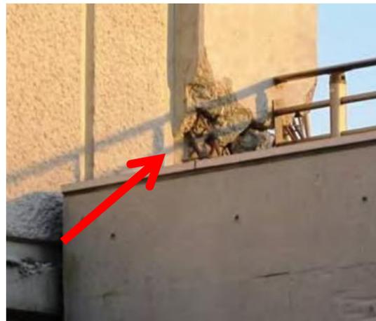
**Figure 2-22: Crushing at the base of the RC column (modified from: Nishiyama et al., 2011).**
