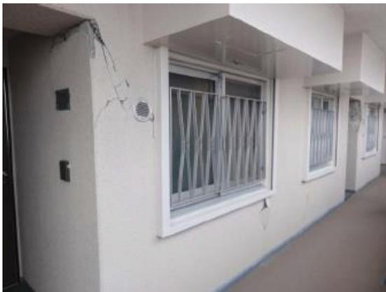
Figure 2-17: Damage to reinforced concrete building in Sendai - example 2 (Ventura, 2011).
