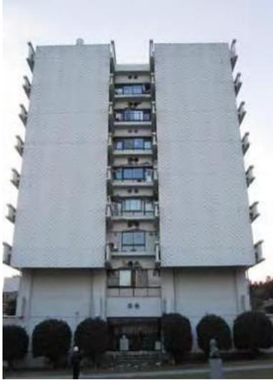
**Figure 2-23: Elevation view of the 8-storey shear wall building in Sendai (Nishiyama et al., 2011).**
