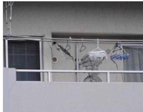
Figure 2-16: Damage to reinforced concrete walls in Sendai - example 1 (Ventura, 2011).
