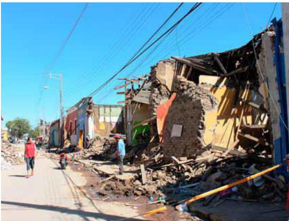
**Figure 2-5: Damage to masonry low-rise buildings in Talca, Maule region (EERI, 2010).**
