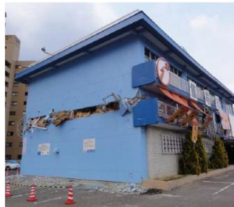
Figure 2-18: Collapse of a mid-story of a reinforced concrete building in Sendai (Ventura, 2011).
