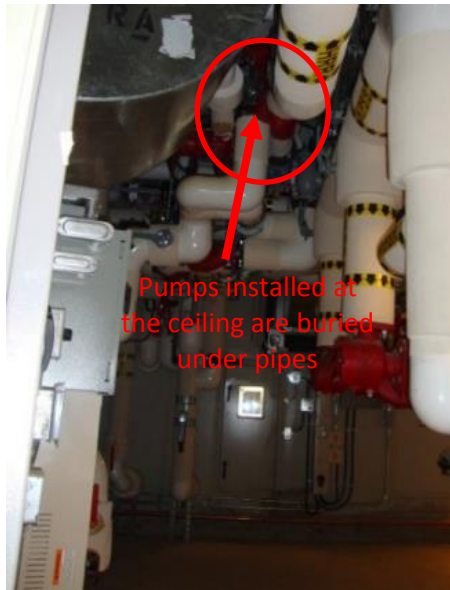
Figure 32: Model queries developed from the owner’s design requirements for mechanical equipment accessibility help timely identification of design characteristics that effect maintenance performance before the start of the operations phase
