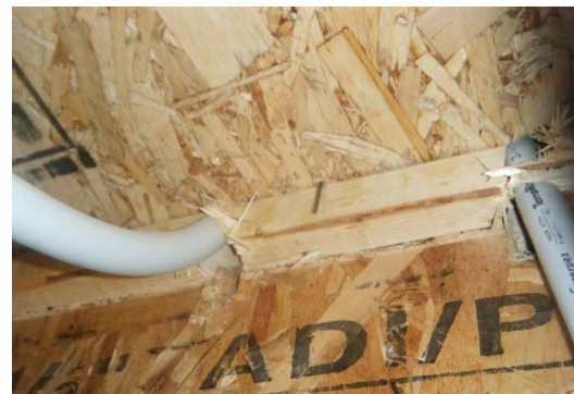
Flange Notched I-Joists
