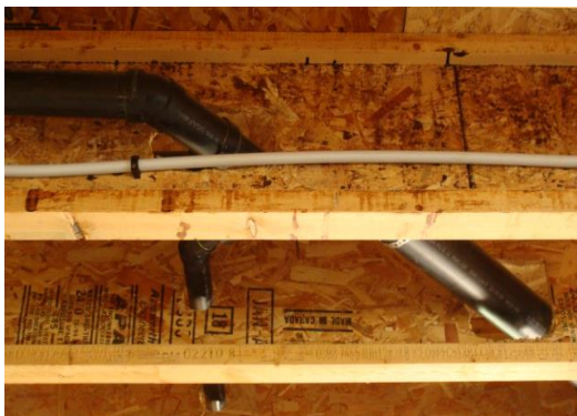
Flange Notched I-Joists
