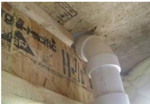
Flange Notched I-Joists
