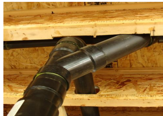
Web Holed I-joists
