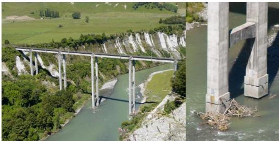
**Figure 2.18 South Rangitikei Rail Bridge with a close up of the rocking piers [from Ma (2010a)]**
