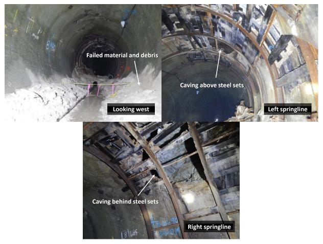
Figure 45: Rock mass at chainage 8+510, showing caving behind the steel sets and the failed debris in the invert.
