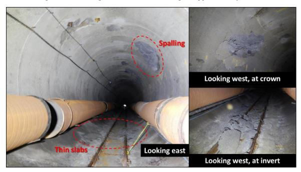
Figure 28: Spalling of rock mass at a chainage of approximately 11+730.
