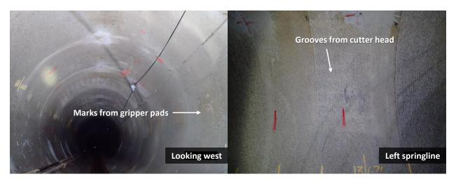
Figure 44: Rock mass at chainage 13+665, showing the grooves and marks left by the TBM.
