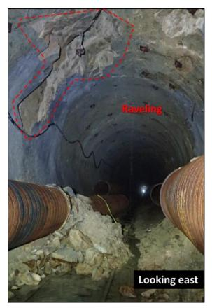
Figure 27: Ravelling of rock mass at a chainage of approximately 8+850.
