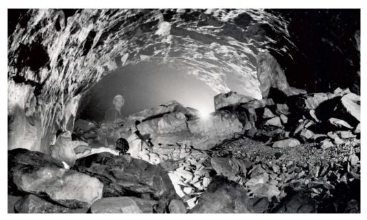
Figure 47: Failure located near chainage 4+700 in the T1 tunnel caused by unstable fault material (HMM, 2010).
