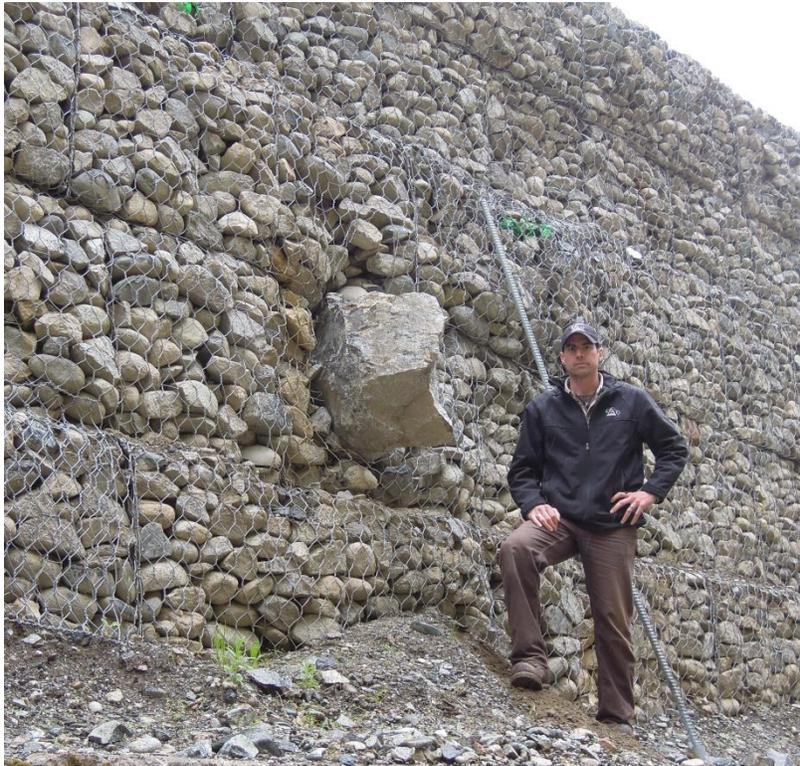
**Figure 4.3: Example of plastic impact where a rock fall is embedded in a gabion wall**
