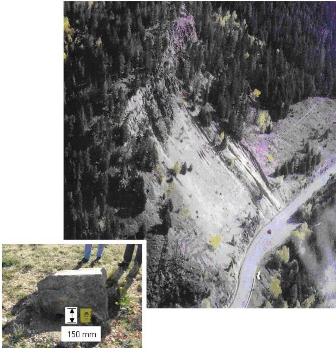
Figure 2.9: View of 138 m (450 ft) high slope comprising 58 m (190 ft) high rock slope where rock fall originated, colluvium slope at 42 degrees, and 10 m (33 ft) high cut face above the road
