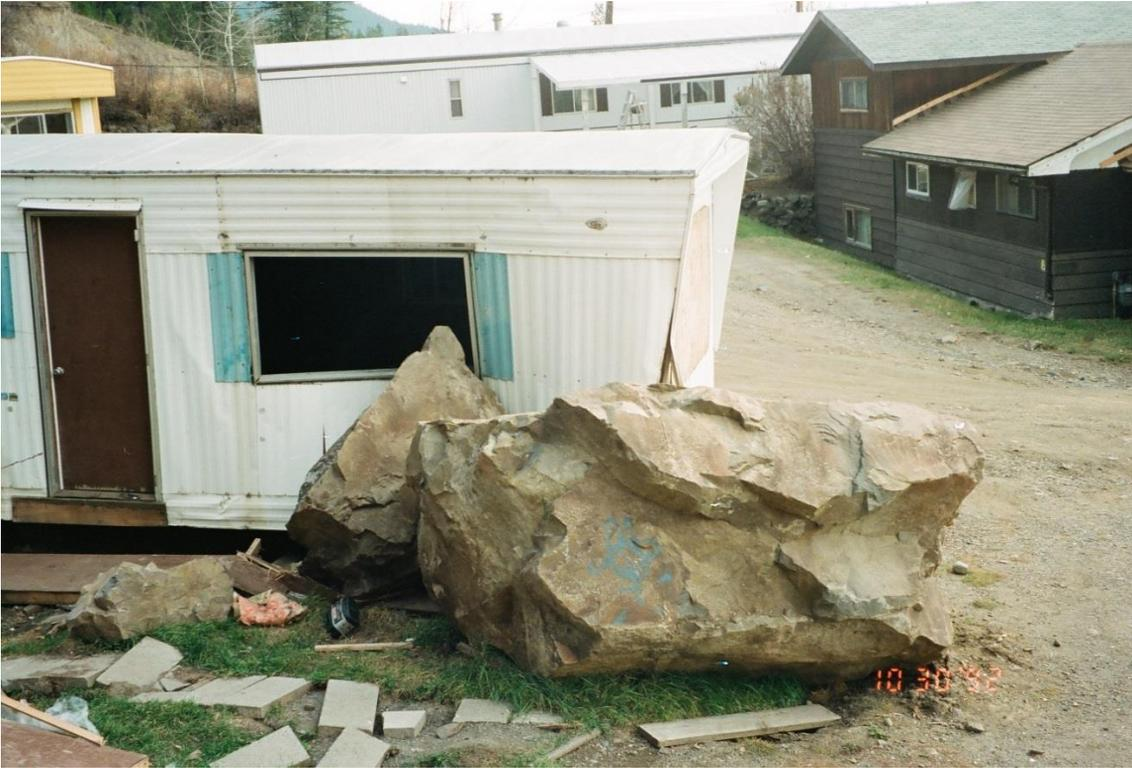
**Figure 6.1: Rock fall that stopped, just before causing serious damage to a building, when it impacted a horizontal surface that absorbed most of the fall energy**
