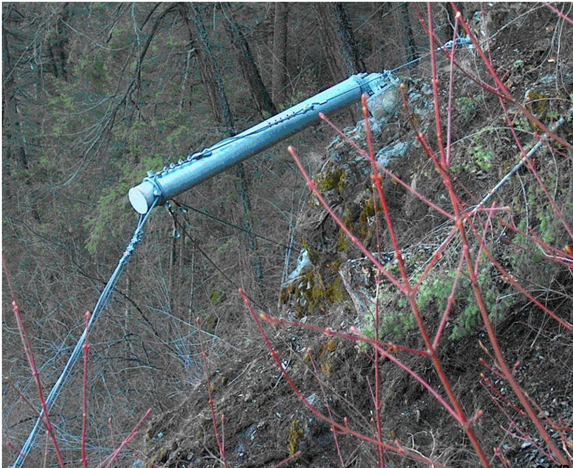
**Figure 8.5: Low friction hinge at base of post allowed the post to deflect, with no damage to the foundation, during an impact that exceeded the service limit states energy (above Shuswap Lake, British Columbia, Canada)**
