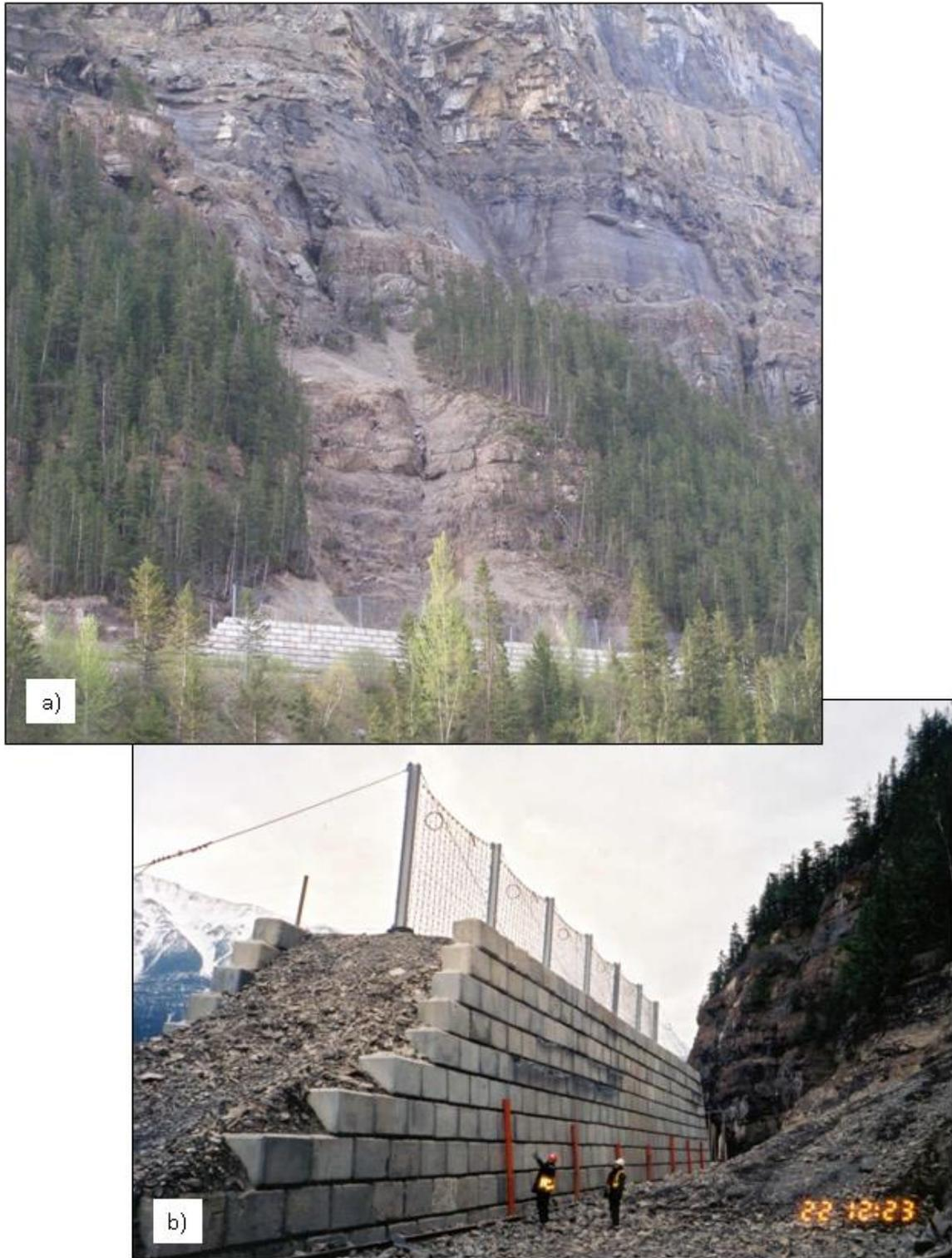
**Figure 2.1: Mt. Stephen rock fall site. a) view of lower third, approximately, of rock face with concrete block barrier at base of slope; b) MSE barrier constructed with concrete blocks, compacted rock fill and Geogrid reinforcing strips, with steel mesh fence along top, to contain rock falls and snow avalanches (courtesy Canadian Pacific Railway)**
