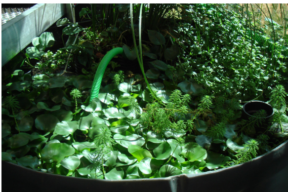
Fig. 3.17. Aerobic tanks. Solar Aquatics System™. CIRS Building, UBC Vancouver campus, Canada.
