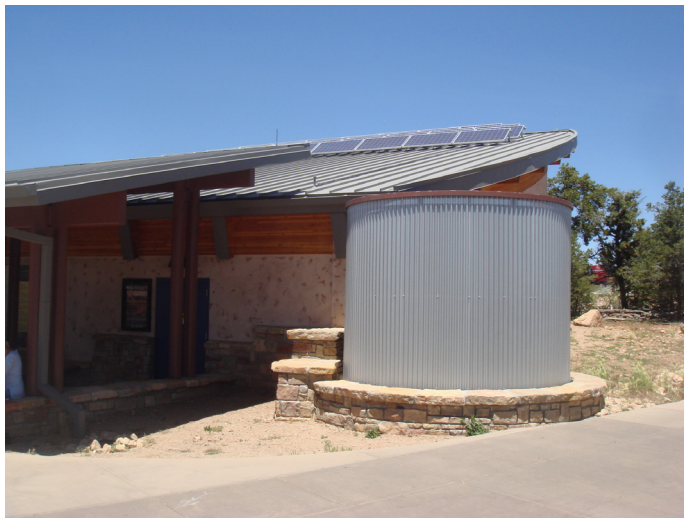
Fig. 3.1. Rainwater harvesting system. Grand Canyon National Park, South Rim visitor center. Arizona, USA.
