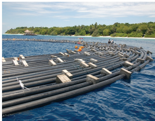
Fig. 5.17. Soneva resort, deep sea water cooling system. Source: Soneva
