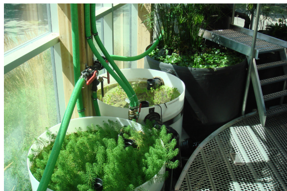
Fig. 3.18. Gravity clarifiers. Solar Aquatics System™. CIRS Building, UBC Vancouver campus, Canada.
