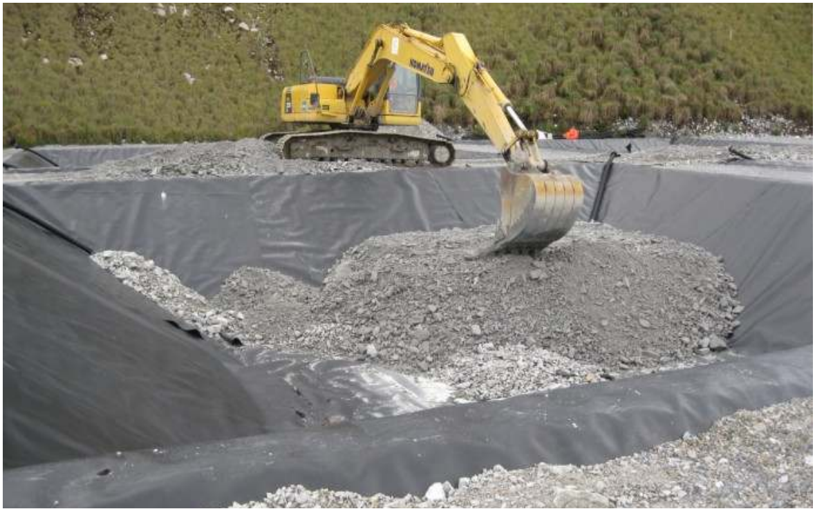
Photo #24: Class A Intrusive placed in lysimeter #1 by excavator.
