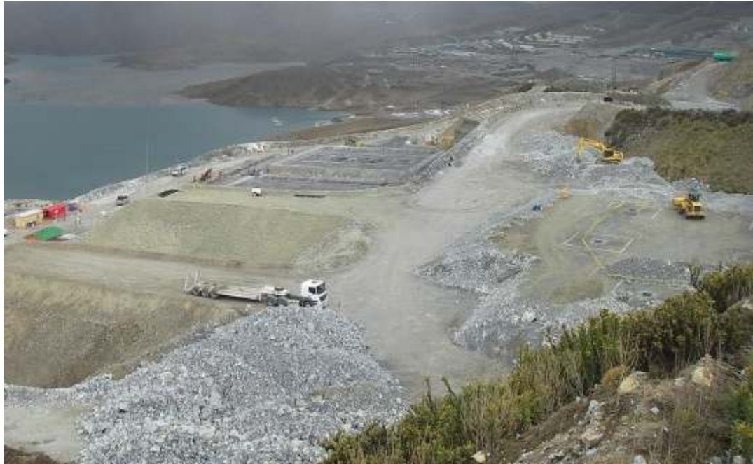
Photo #8: Building the sloped walls of the lysimeters.
