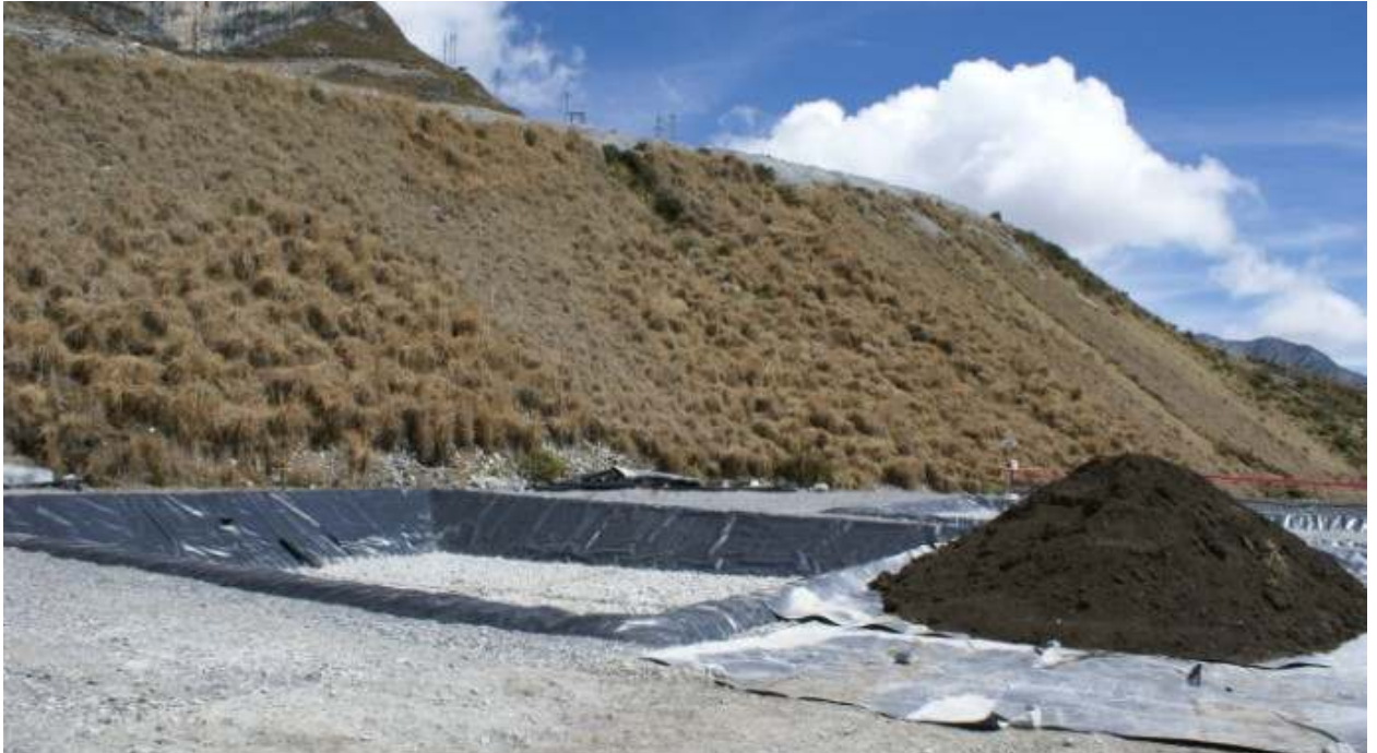
Photo #30: Placing topsoil cover in lysimeter #4.
