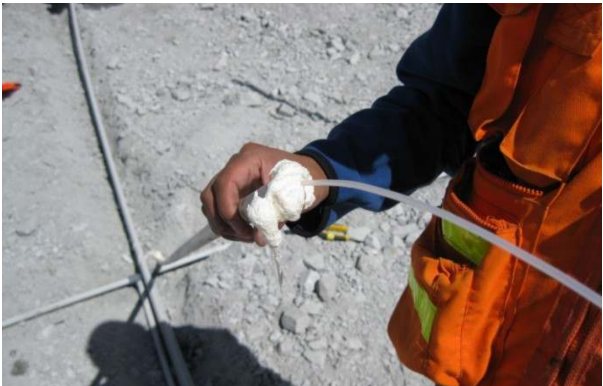
Photo #81: Sealing PVC pipes with expandable foam (see oxygen sampling tube inside).
