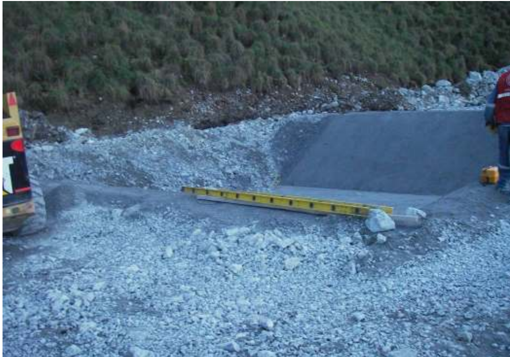
Photo #10: Bituminous liner installation on the lysimeters.
