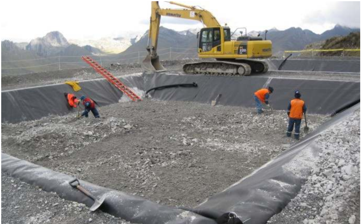
Photo #26: Class A Intrusive already leveled in lysimeter #2.
