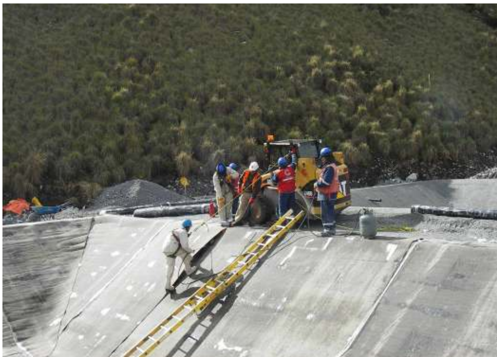
Photo #10: Bituminous liner installation on the lysimeters.
