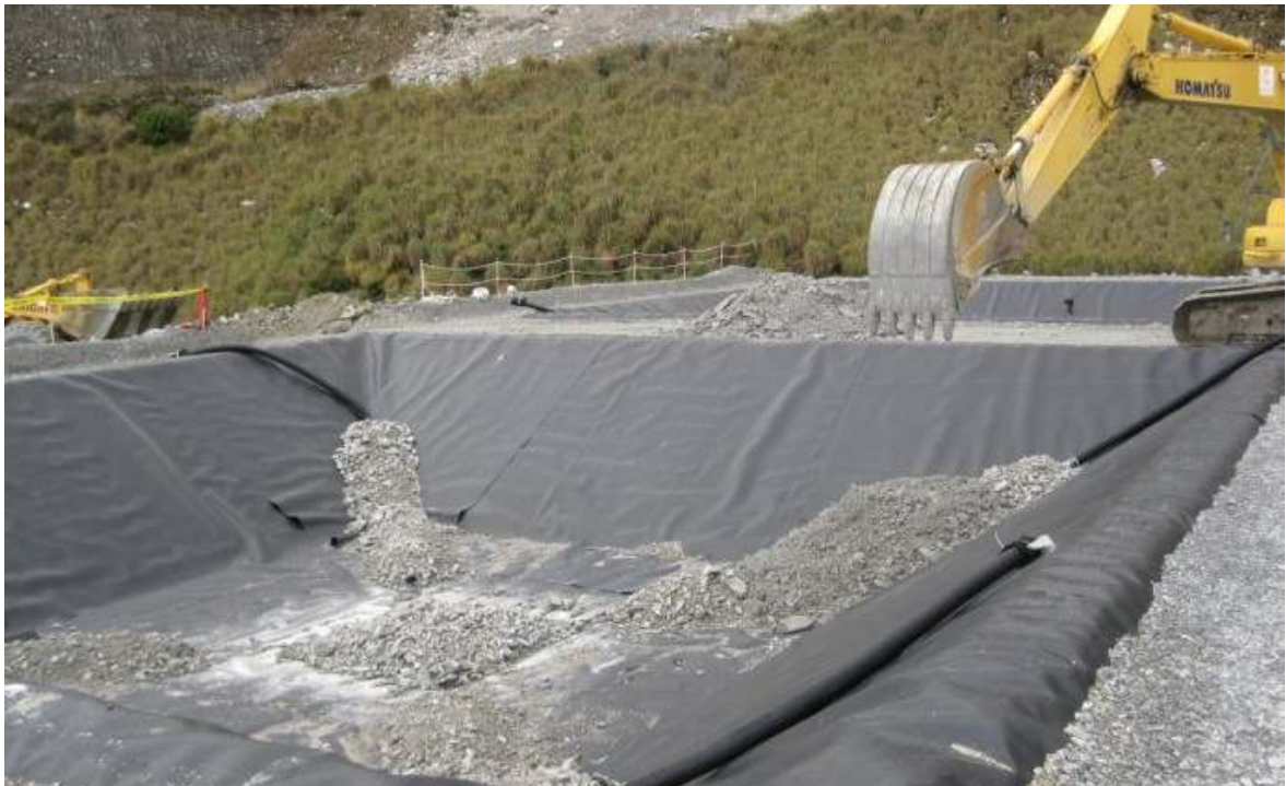
Photo #22: Placing Class A Intrusive in lysimeter #5.
