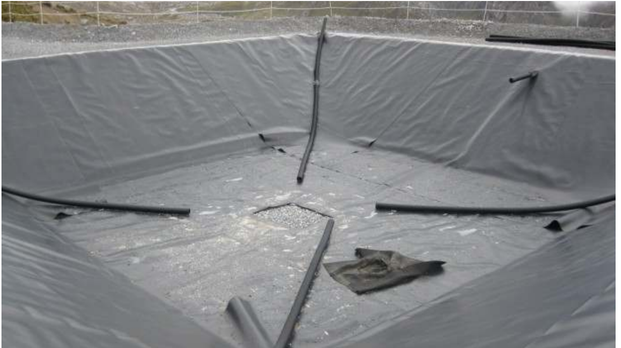
Photo #18: Part of the already built sump excavated and geotextile placed for the construction of the new filter.
