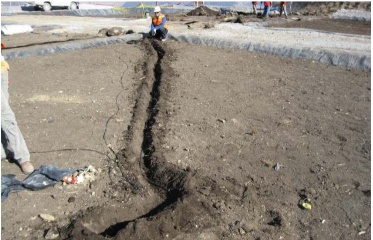
Photo #77: Trench in topsoil cover for taking TC sensors cables to one of the corners of lysimeter #2.
