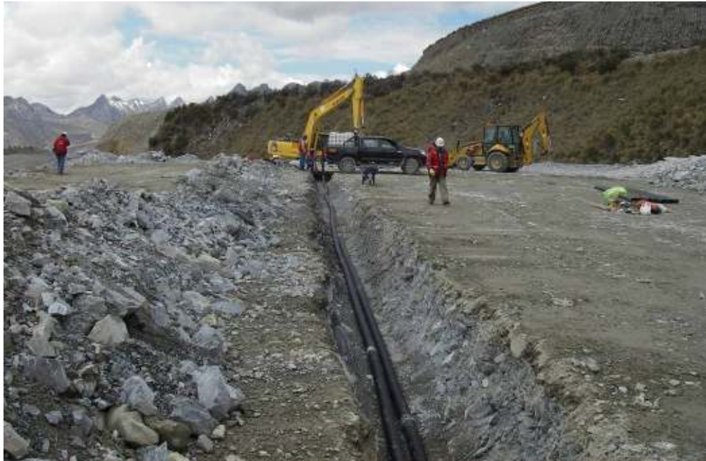
Photo #6: Sump for infiltration piping system, prior the construction of the lysimeter.
