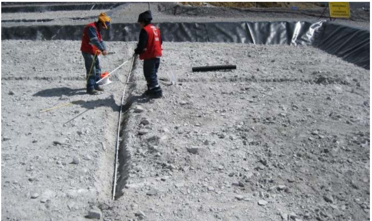
Photo #79: Placing PVC pipes for protecting oxygen sampling tubes.
