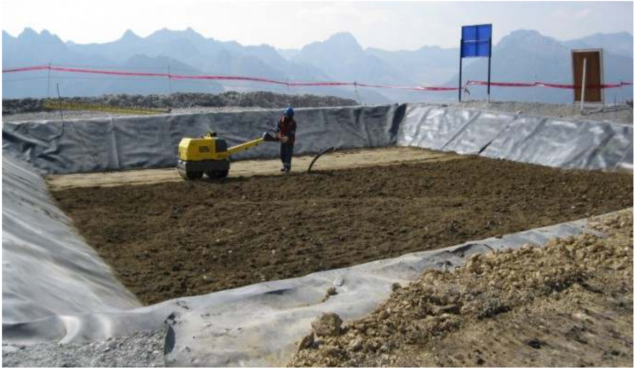
Photo #42: Compacting clayey till in lysimeter #1.
