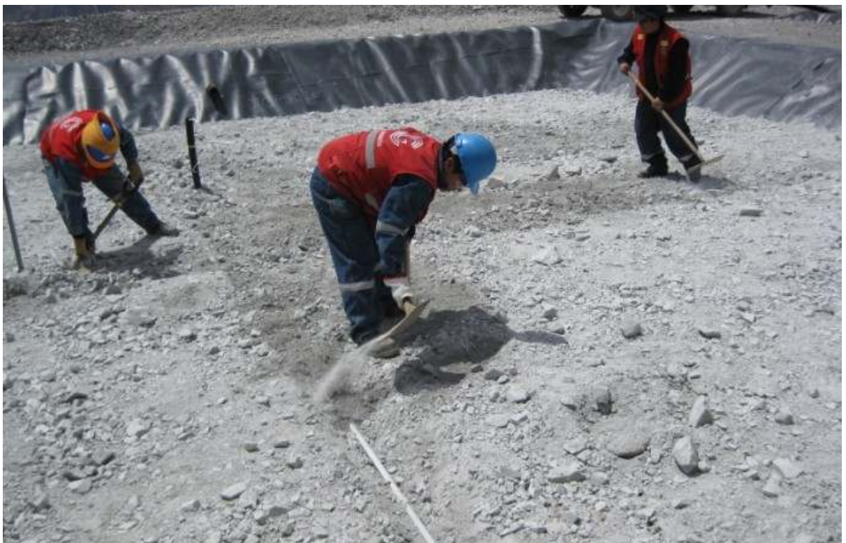
Photo #83: Covering PVC pipes with fine sand for protection purposes.
