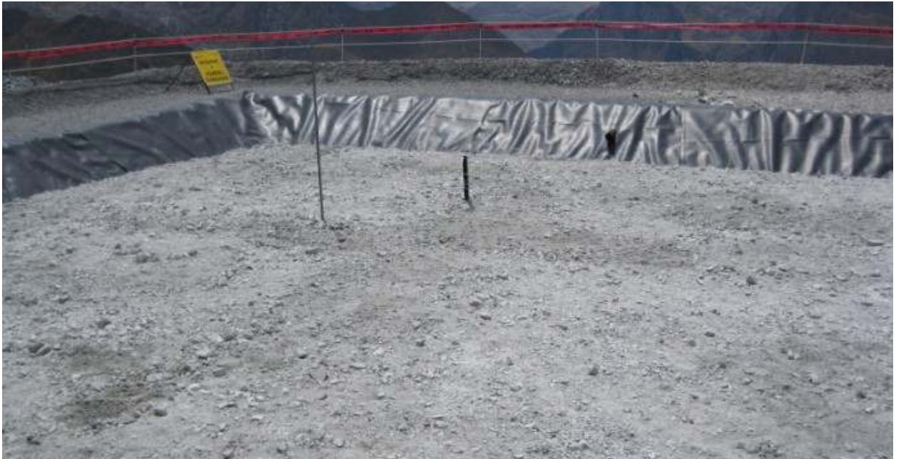
Photo #85: Oxygen sampling tubes coming out of the cover system through HDPE pipe.
