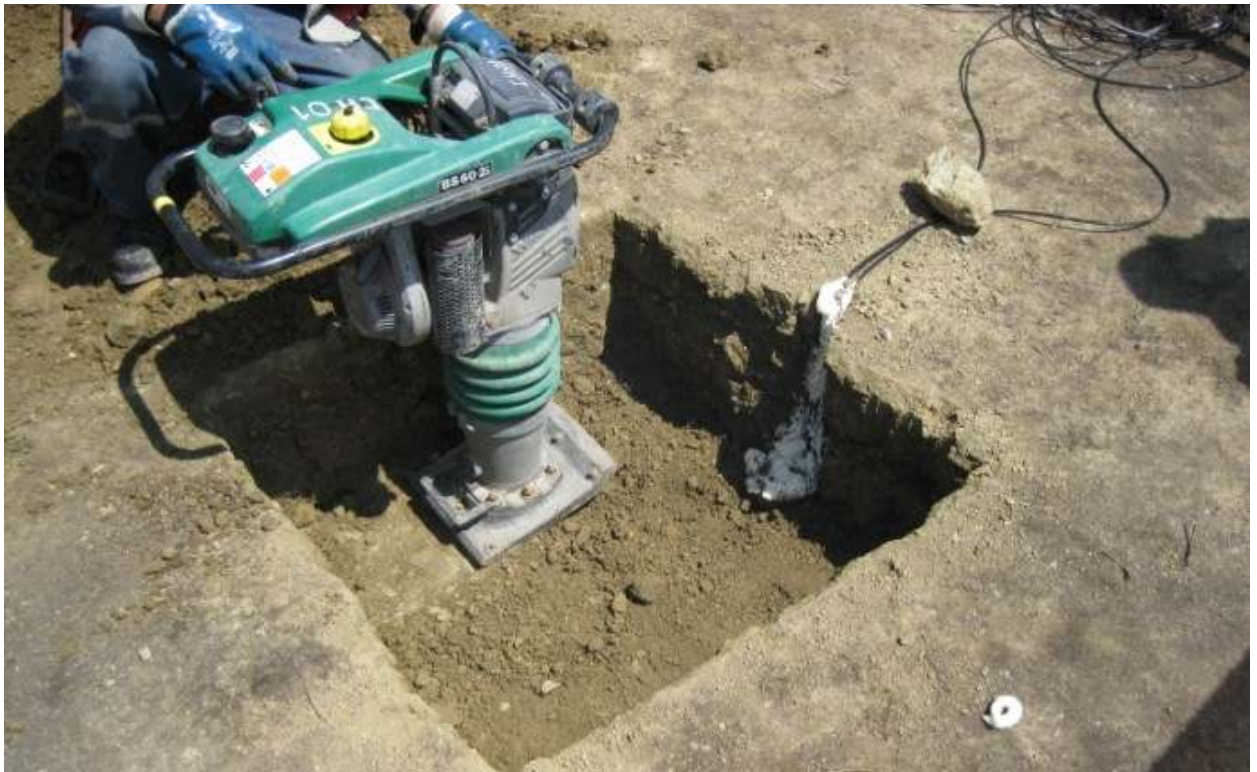
Photo #73: Test pit for installing TC sensors in lysimeter #2.
