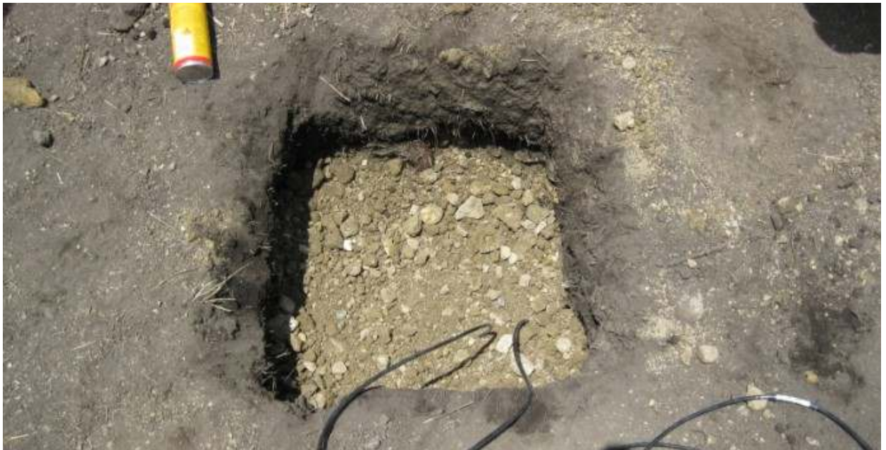
Photo #77: Trench in topsoil cover for taking TC sensors cables to one of the corners of lysimeter #2.
