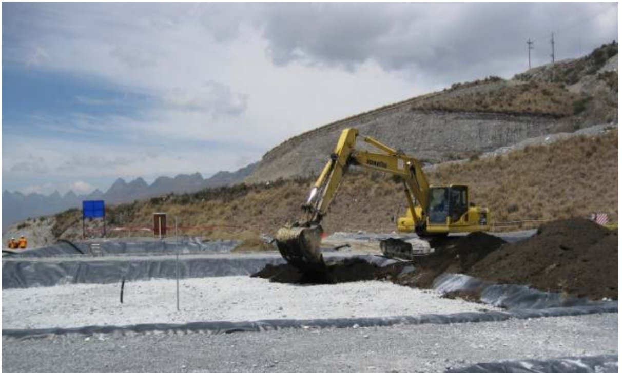
Photo #30: Placing topsoil cover in lysimeter #4.
