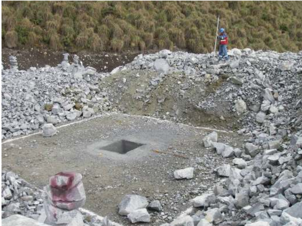
Photo #8: Building the sloped walls of the lysimeters.
