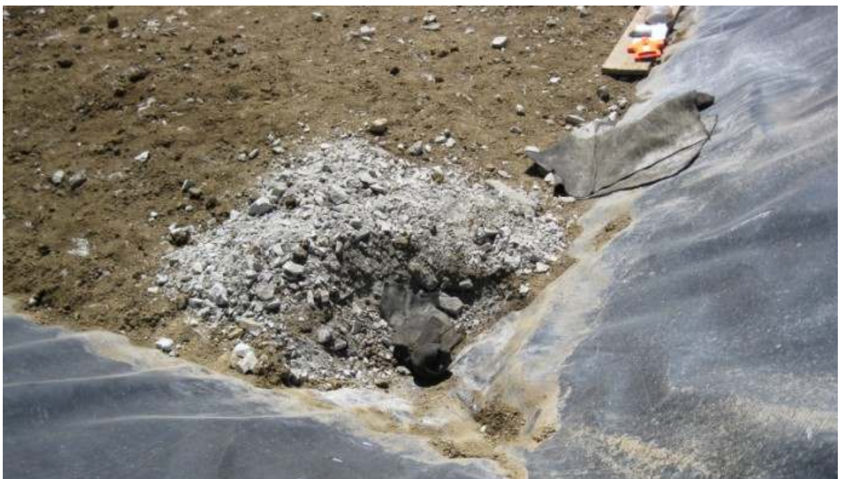
Photo #28: Oxygen pipe cut and capped with geotextile, below Class A Intrusive level.
