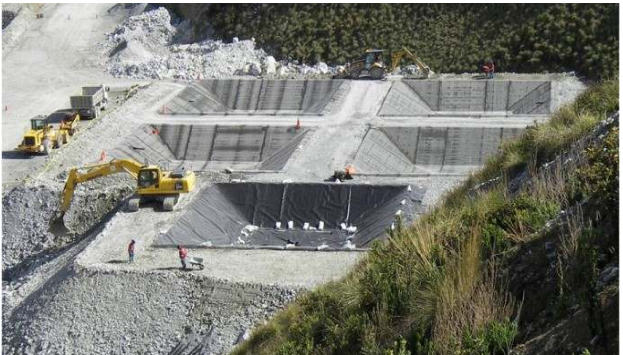
Photo #14: Installing liner in the lysimeters.
