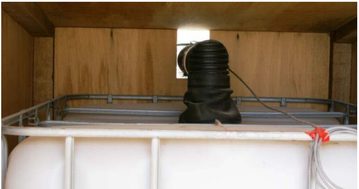
Photo #56: Runoff pipe connection with tank.
