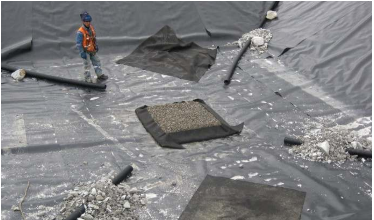
Photo #20: New filter already built geotextile and oxygen pipes fixed with Class A Intrusive material.
