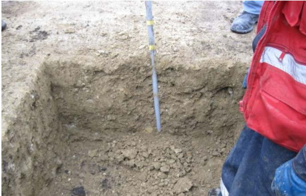
Photo #63: Horizontal PVC pipes left in the cover system to get a hole for TC sensors.
