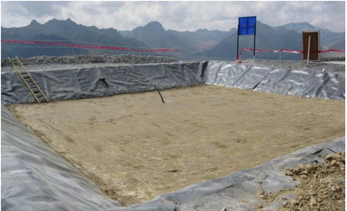
Photo #46: Silty till layer already compacted in lysimeter #5.
