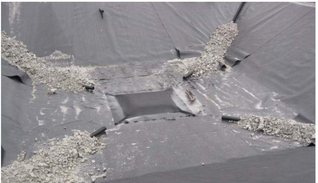
Photo #20: New filter already built geotextile and oxygen pipes fixed with Class A Intrusive material.
