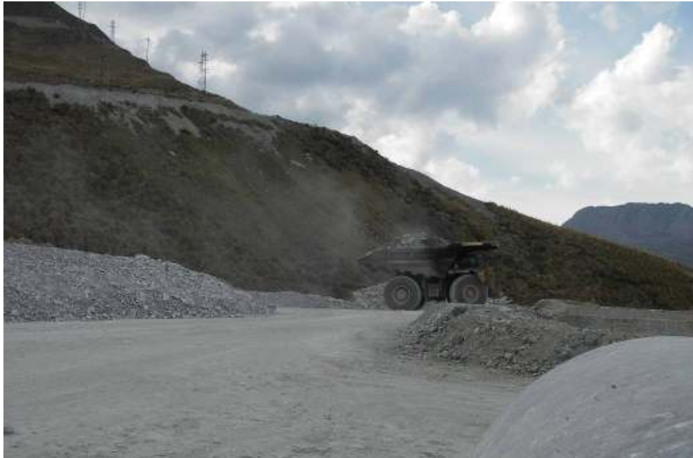
Photo #4: Compacting placed material for the base of the lysimeters.
