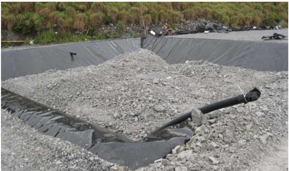
Photo #24: Class A Intrusive placed in lysimeter #1 by excavator.
