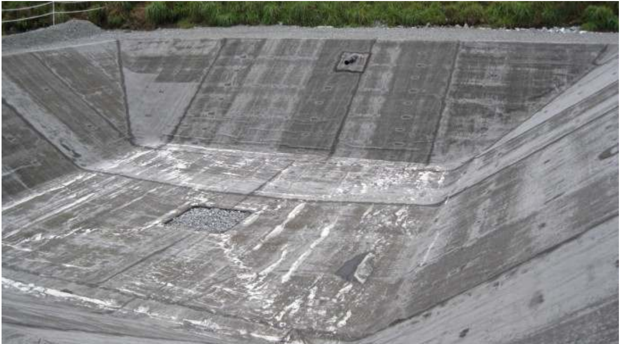
Photo #14: Installing liner in the lysimeters.
