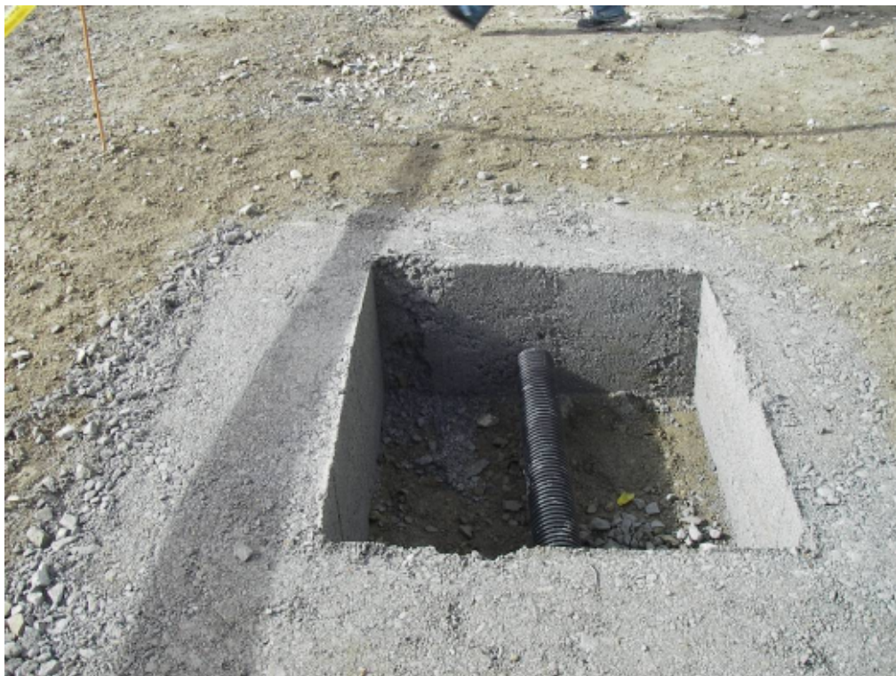
Photo #6: Sump for infiltration piping system, prior the construction of the lysimeter.
