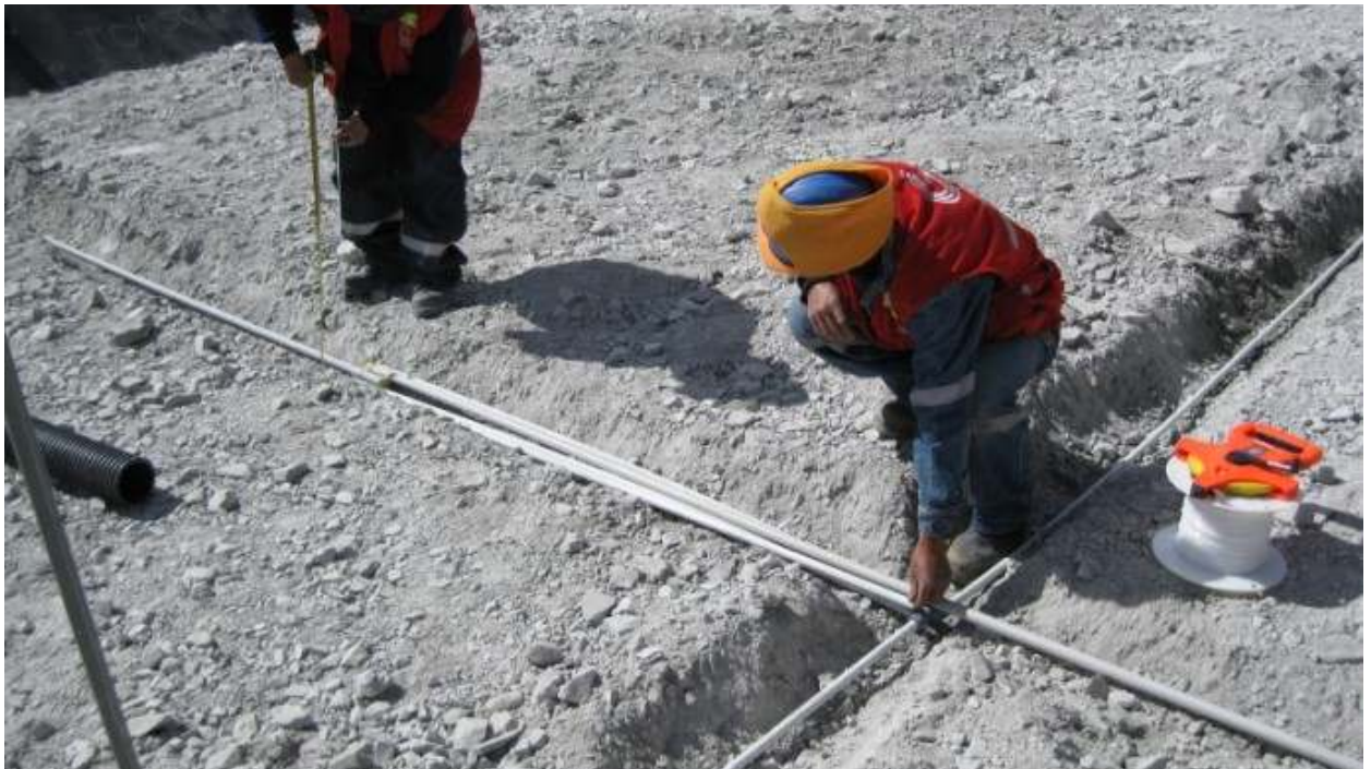
Photo #81: Sealing PVC pipes with expandable foam (see oxygen sampling tube inside).
