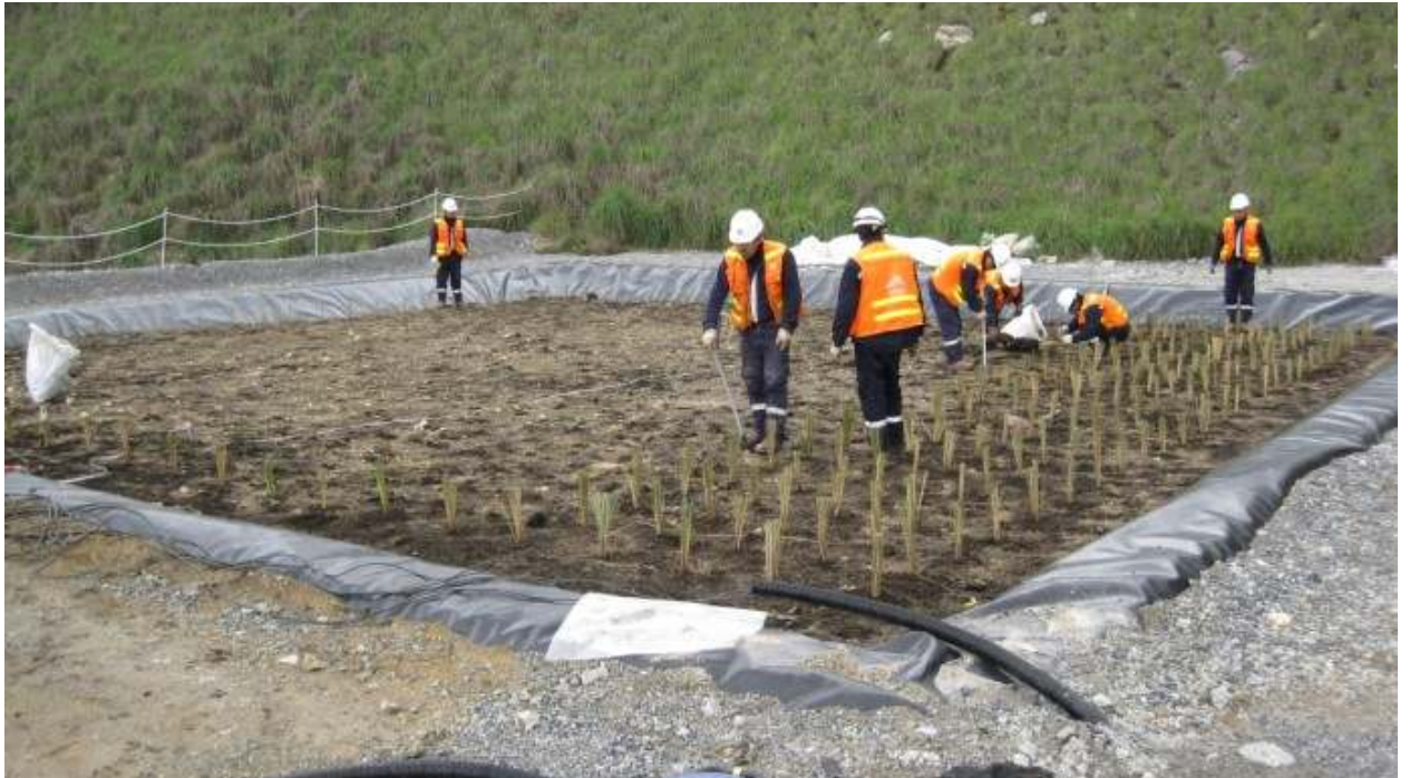
Photo #88: Transplanting Calamagrostis sp. (locally known as Ichu) to topsoil cover.
