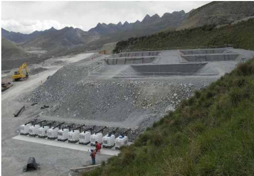
Photo #16: Lysimeters, piping and tanks completed.
