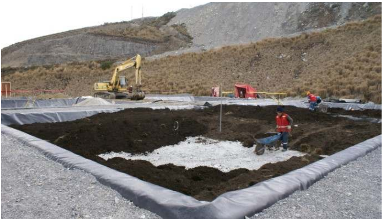
Photo #32: Building topsoil cover in lysimeter #4.
