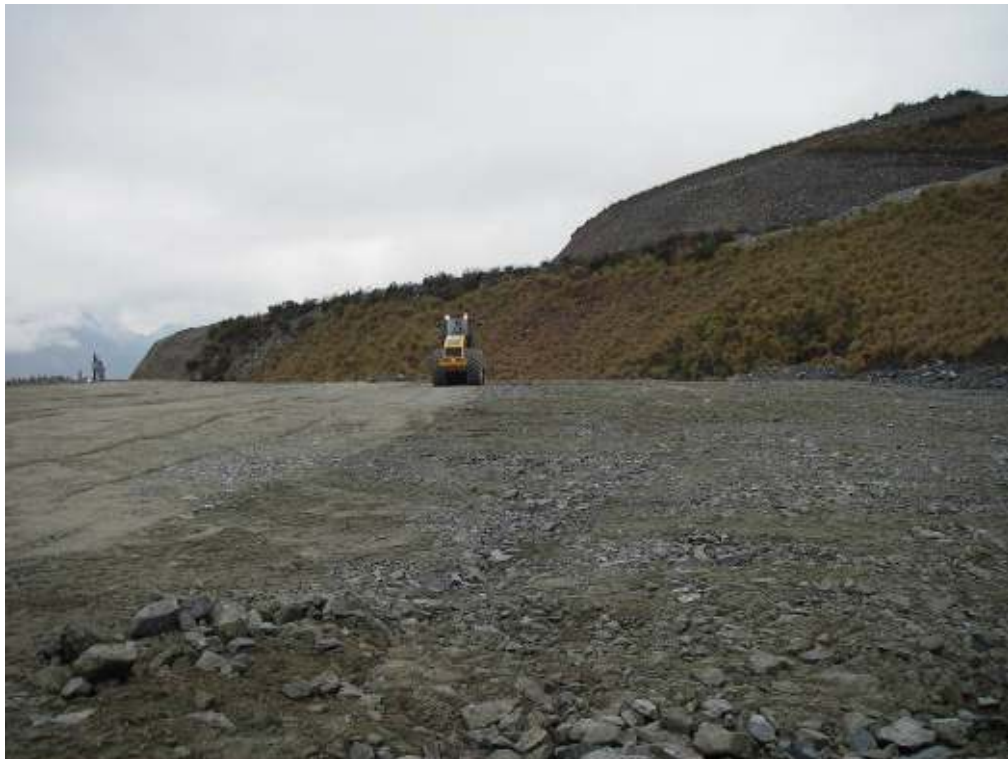
Photo #4: Compacting placed material for the base of the lysimeters.
