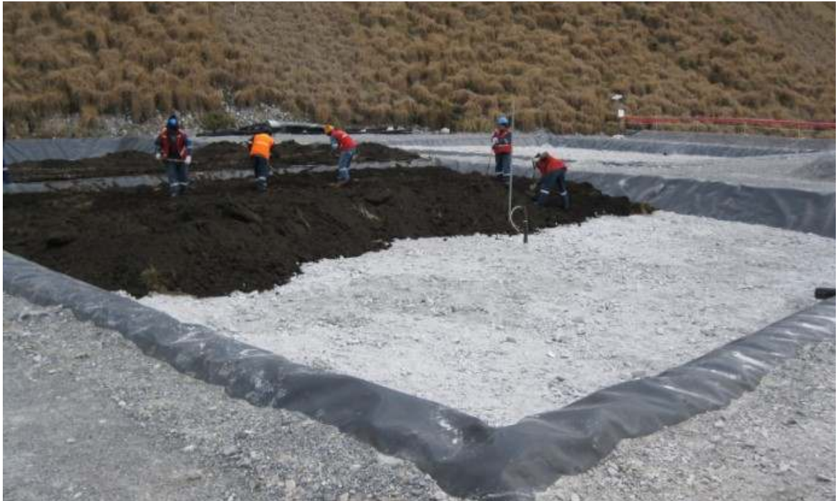
Photo #32: Building topsoil cover in lysimeter #4.
