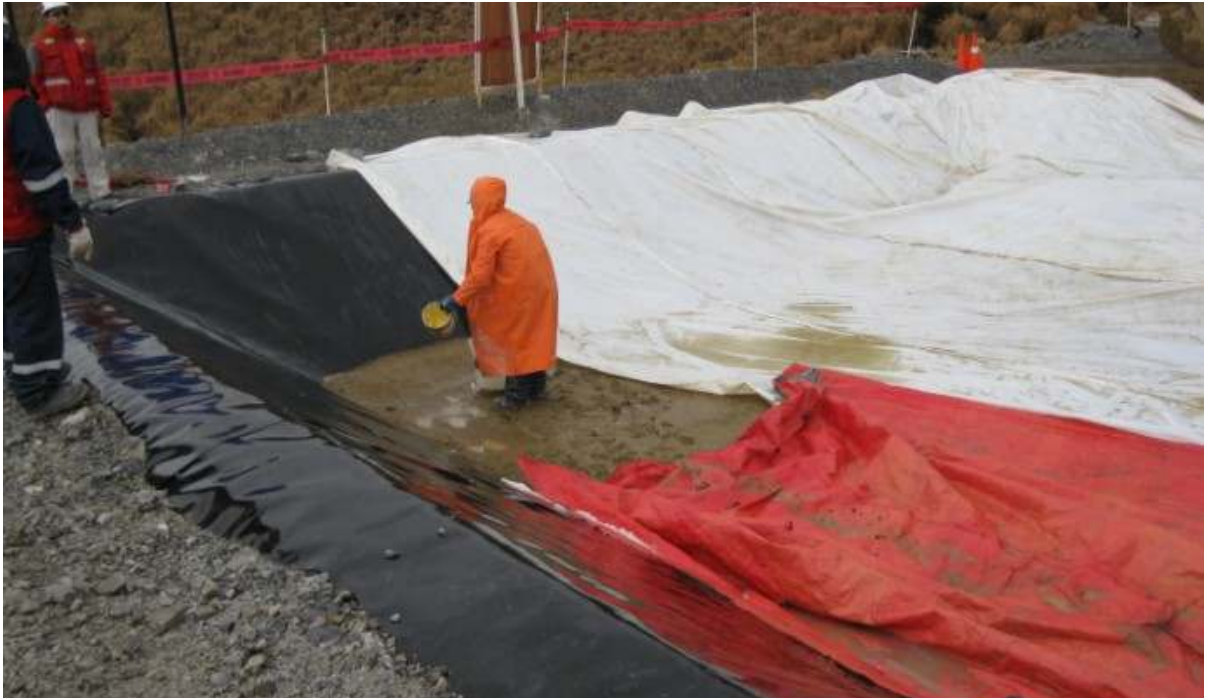
Photo #46: Silty till layer already compacted in lysimeter #5.
