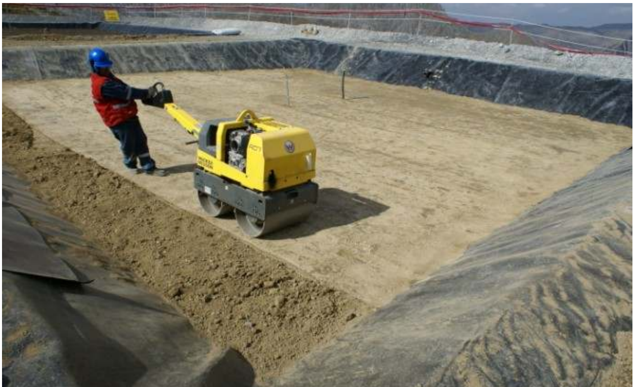
Photo #42: Compacting clayey till in lysimeter #1.
