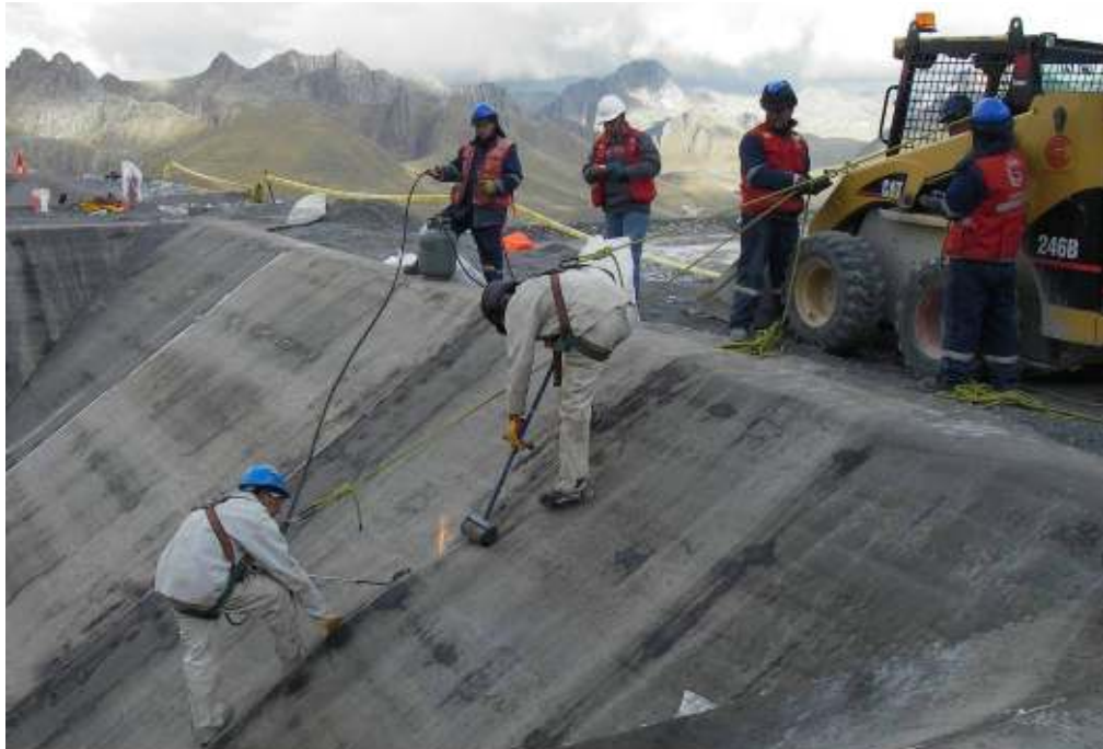
Photo #12: Lysimeter #2 with bituminous liner and run-off and infiltration piping systems already installed.
