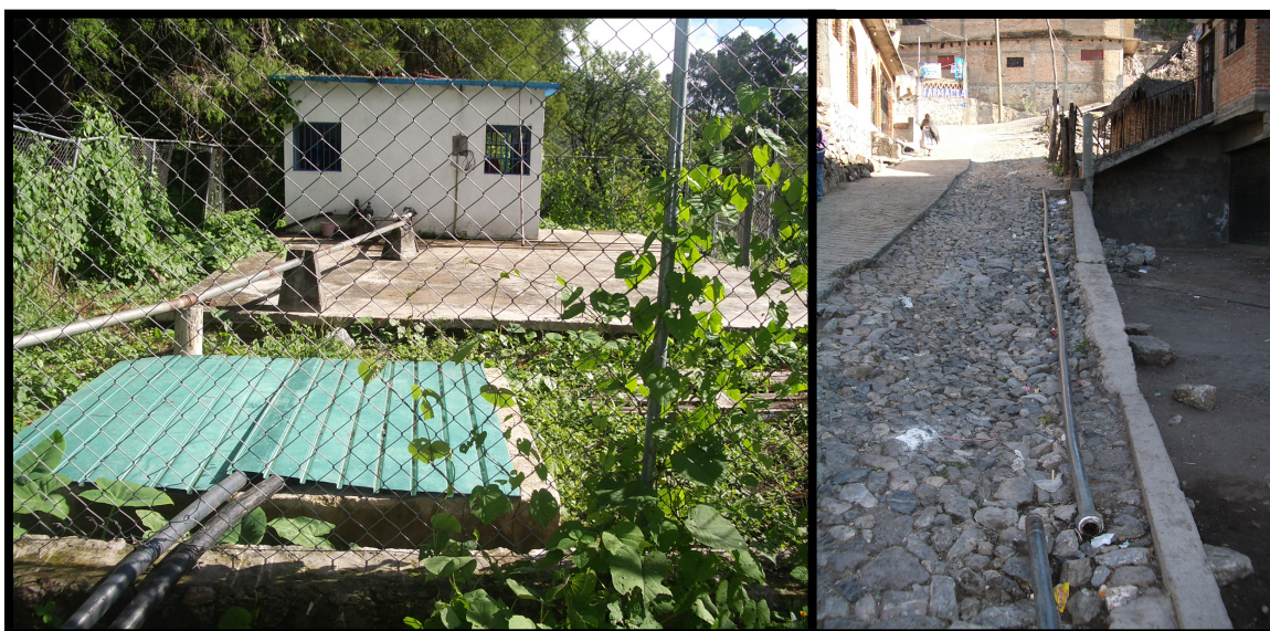
Figure 3.9 (a) Pumping station located at Los Sabinos (b) Broken distribution pipes
