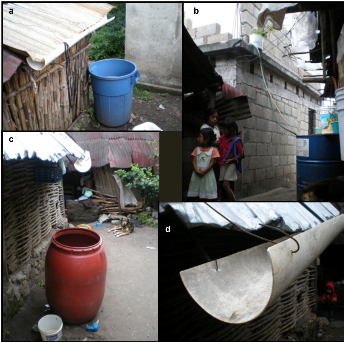
FIGURE 3.7 EXAMPLES FROM 4 PARTICIPANT HOUSEHOLDS OF TUBING AND HOSES DIRECTING RAINWATER RUNOFF FROM ROOFS TO VARIOUS CONTAINERS
