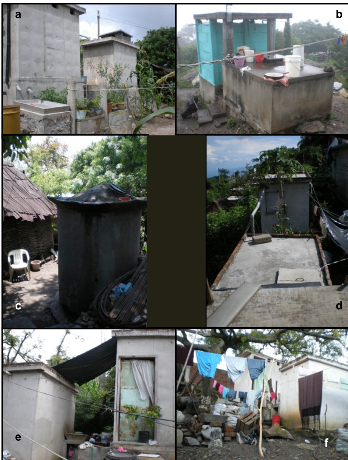
FIGURE 3.8 EXAMPLES FROM SIX PARTICIPANT HOUSEHOLDS OF CISTERNS THAT CAPTURE RAINWATER FROM THEIR OWN ROOFS
